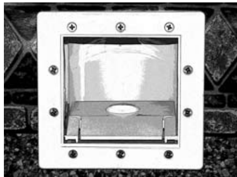
Skimmer faceplate installed.
