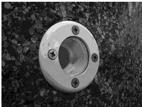
Return faceplate installed.
