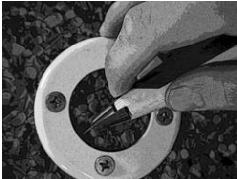
Trim liner from return opening.
