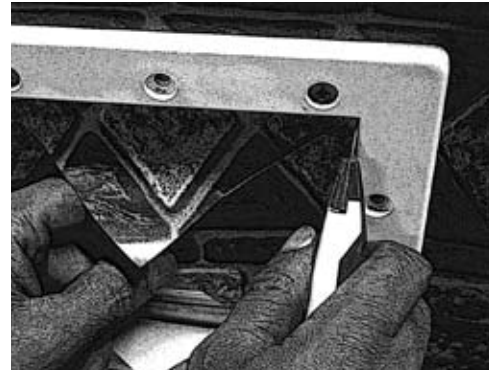
Trim liner from skimmer opening.
