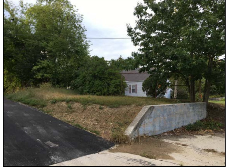
from Homestead Ave, east end of frontage
