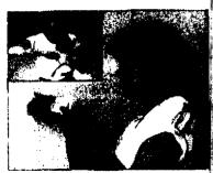
4. Insert the stude into the stud holes on the hade of each letter. Place letters in holes on wall before applying silicone to verify position. Adjust as neces sary. Now fill the deil holes in the wall of the first letter with silicone.
