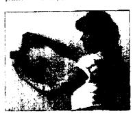
6. Push the letter into the drill holes using a shim to assure the proper standoff of the letter from the wall. Repeat stope 3 through 5 for the rem of the letters.
