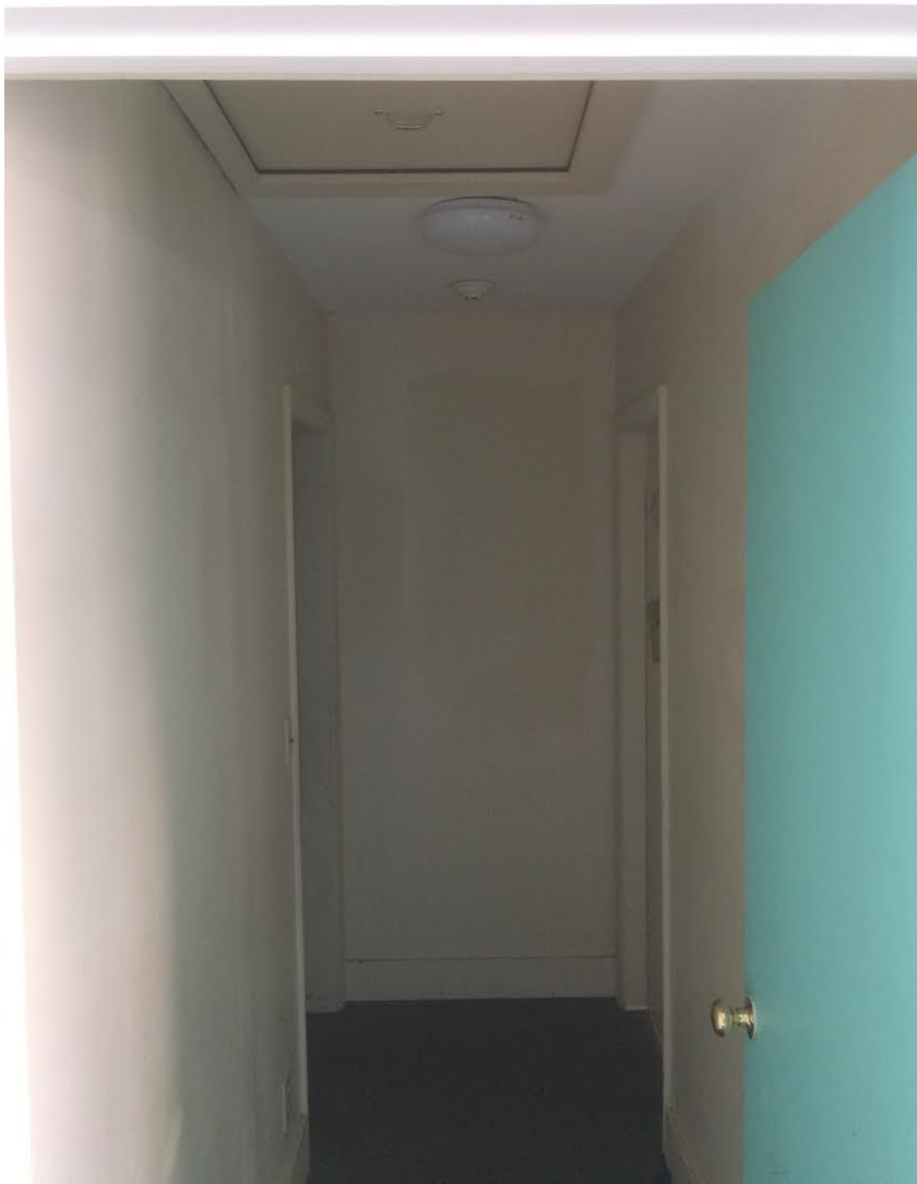
2nd floor corridor with attic access hatch in ceiling
