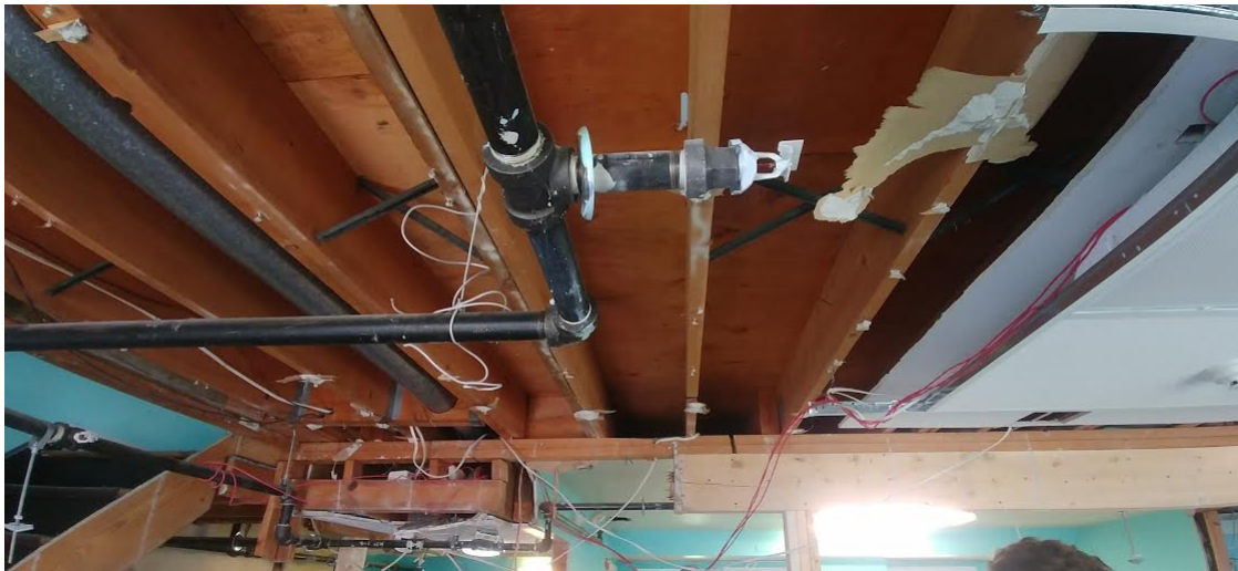
2nd Floor supports, looking up from 1st Floor level
