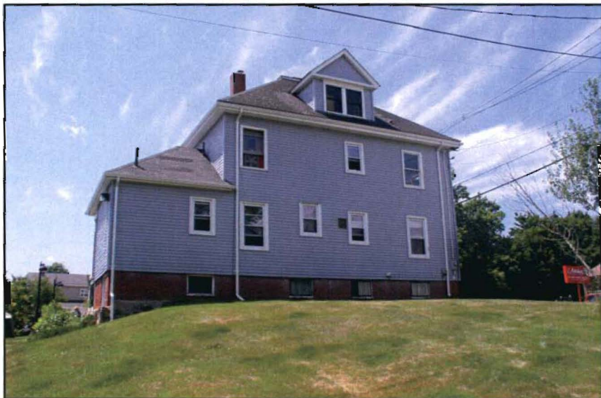
View looking south from Riverside St (top) View of the north side of the residence (bottom)
