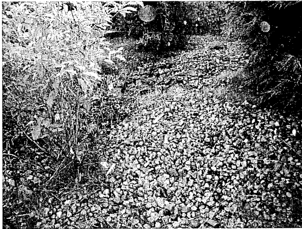
Bioretention Basin Stone Trench Adjacent to Pavement
