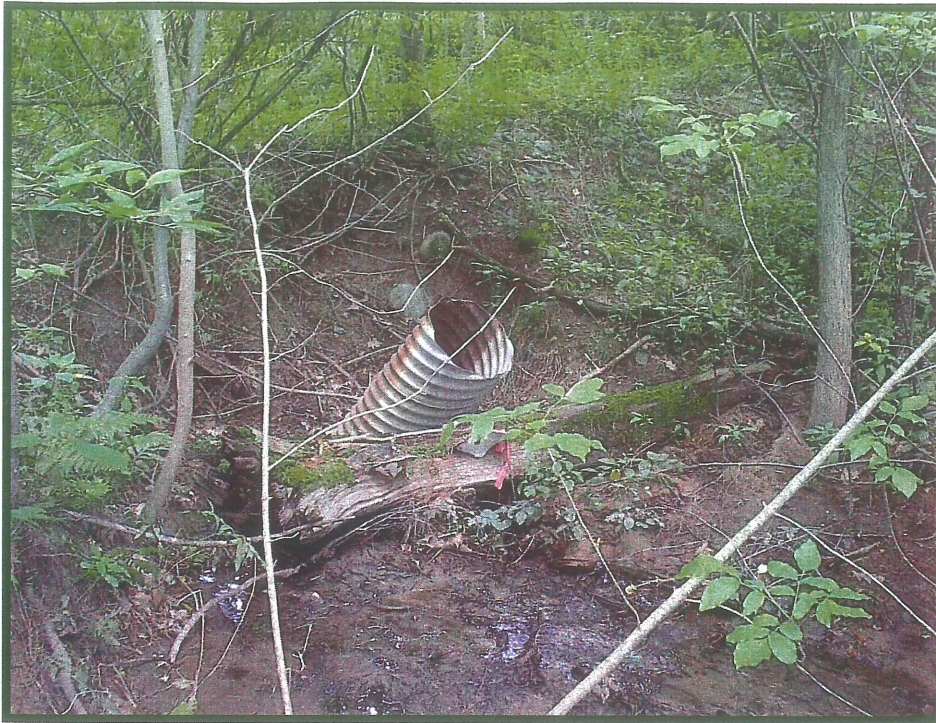
PHOTOGRAPH #5: Looking northerly at exposed culvert in existing stream.
