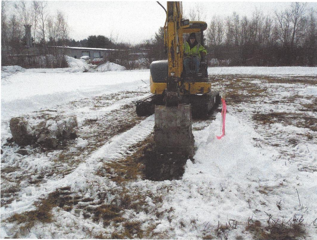
View of excavator near edge of upland
