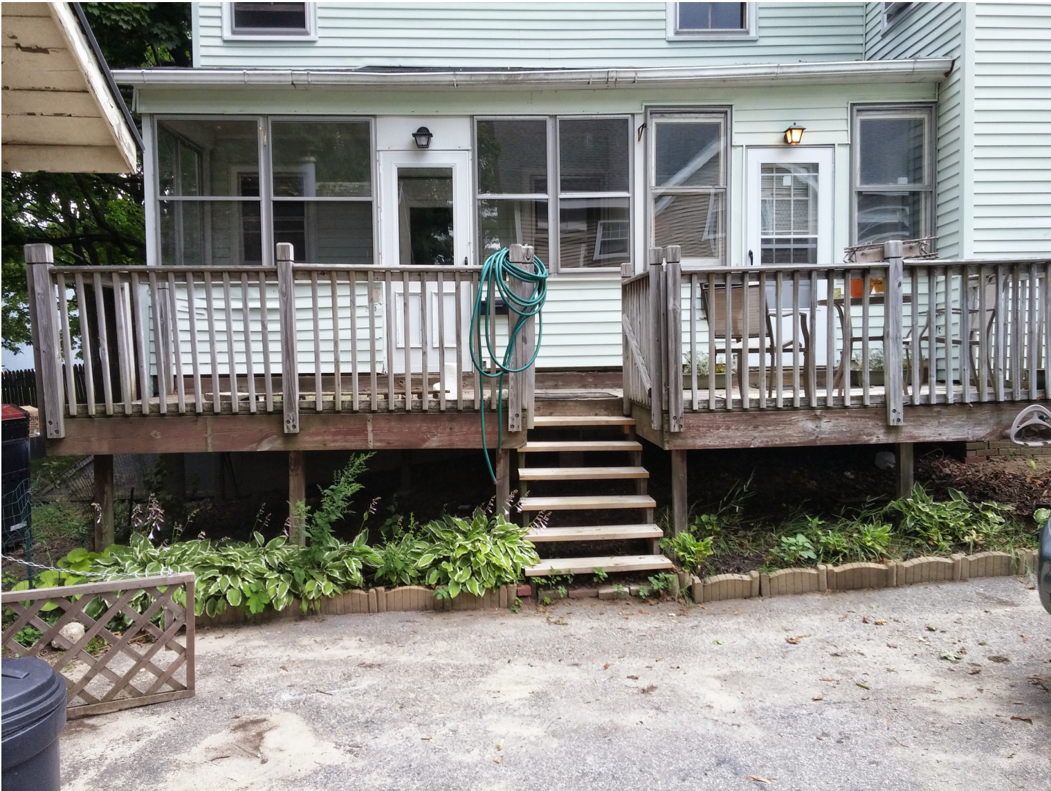
Image of deck to be replaced with stairs.
