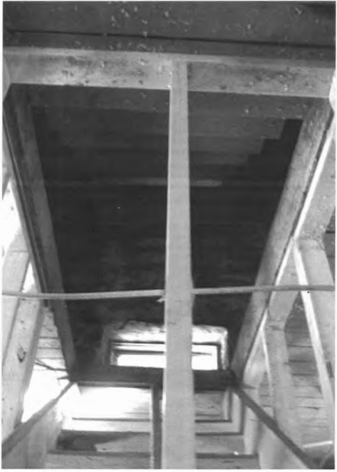
BASEMENT OPENING, (FORMER ACCESS)
