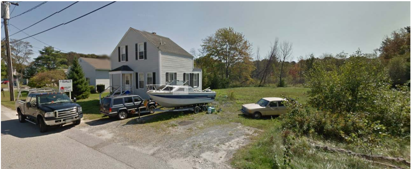
Figure 2: 72 Bishop Street, existing conditions
