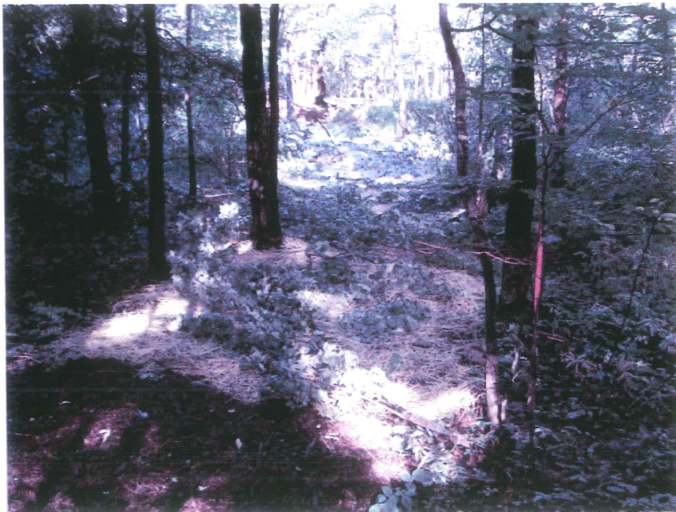
Photograph 4 Westward view across the area where the berm was removed looking toward vantage point of Photo 3.
