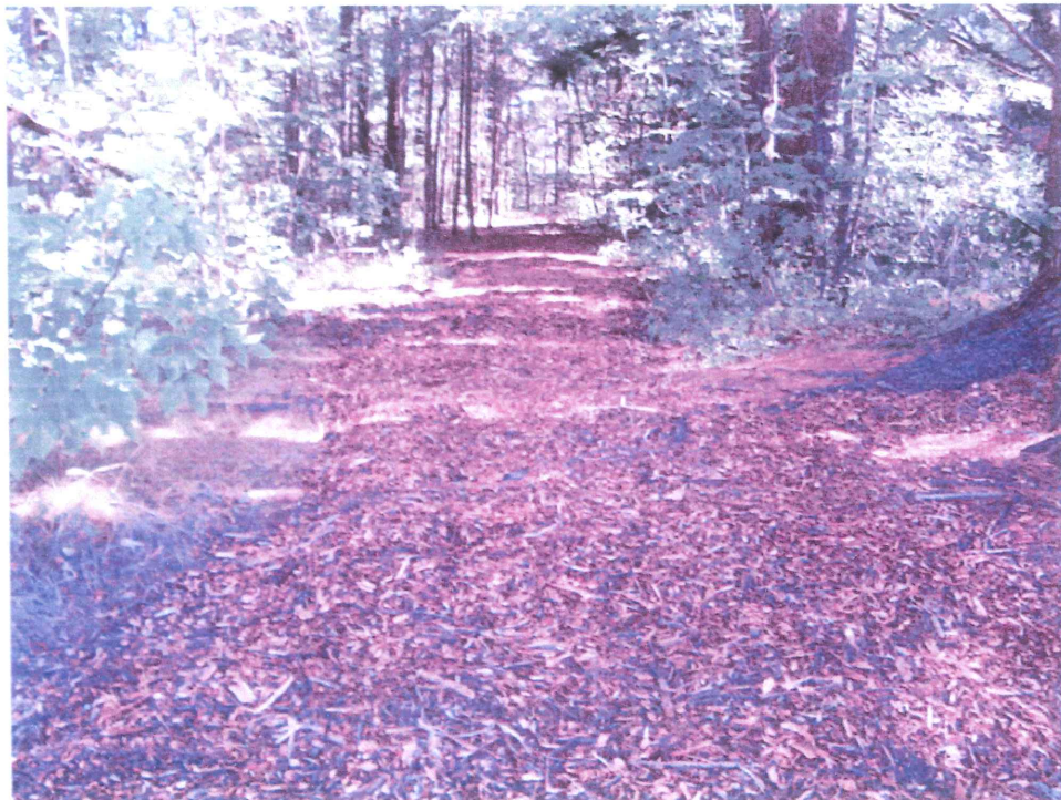
Photograph 6 Northward view of trail between the two new bridges that has been covered with bark mulch to protect eroded, exposed tree roots and improve walking conditions for trail users.
