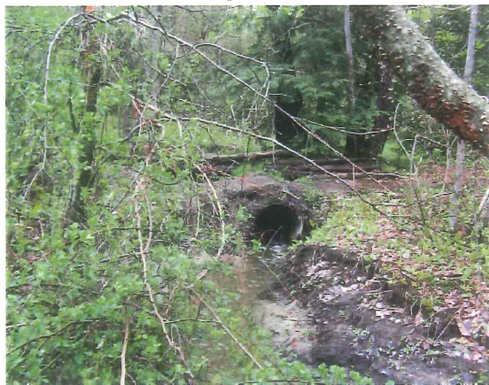
2. Looking southeast at 24-inch culvert.
