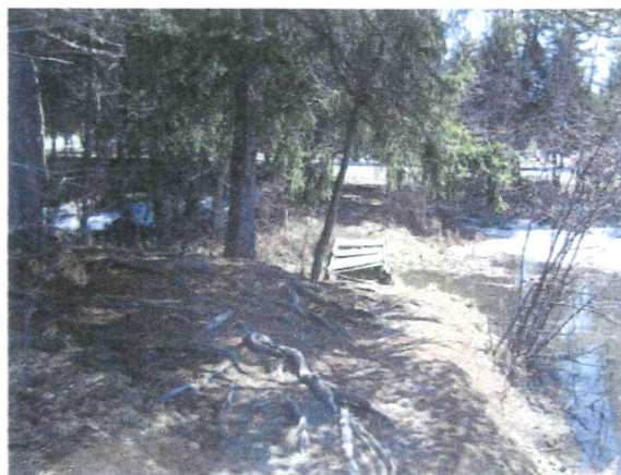
3. Looking southeast at bridge over Pond 1 outlet. ③
