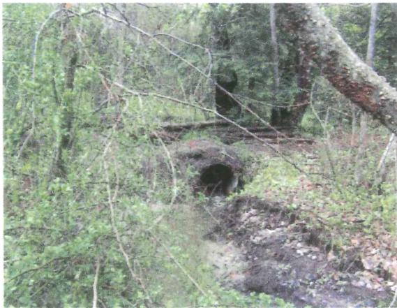
2. Looking southeast at 24-inch culvert. ②
