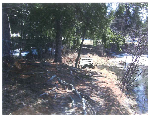
3. Looking southeast at bridge over Pond 1 outlet.
