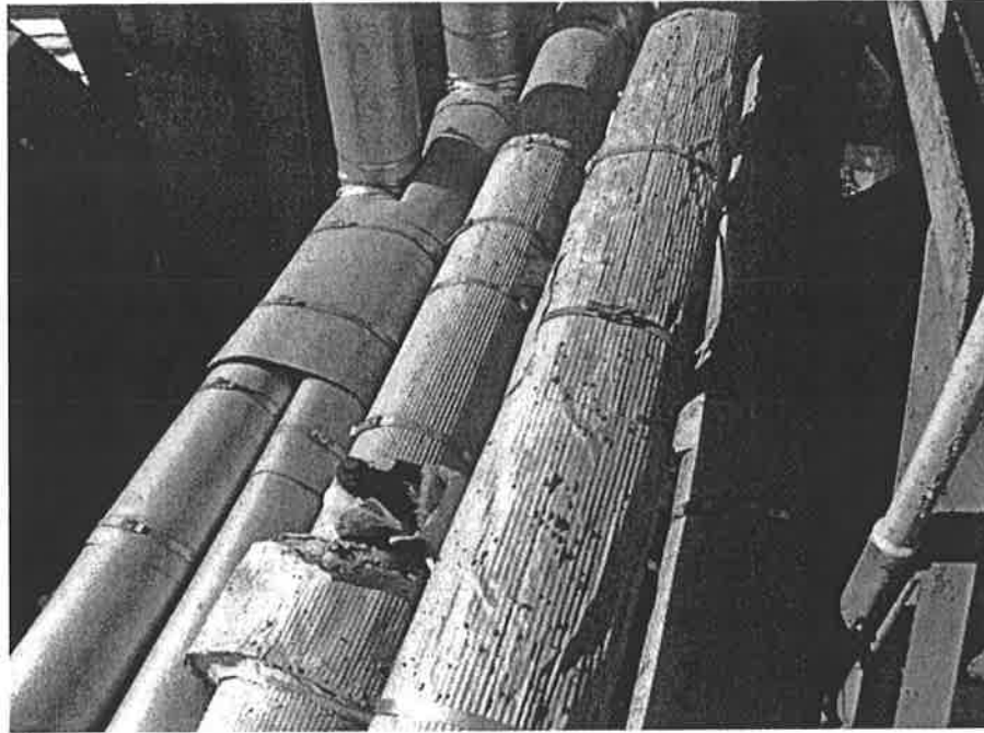
PHOTO 3 Non-ACM pipe insulation in smooth & corrugated aluminum covers
