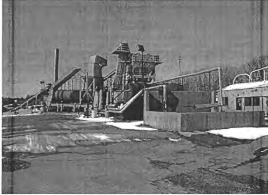
PHOTO 1 Bishop Street Asphalt Plant #910
