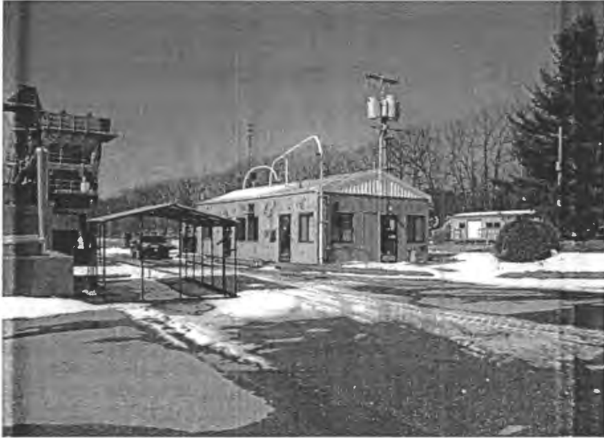
PHOTO 2 Out buildings not included in survey
