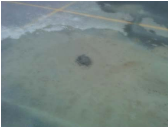
Boring B-3 Location
