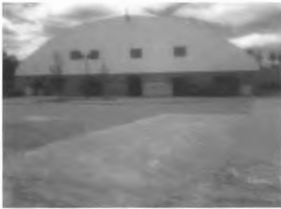
Overall View of Addition Area Facing Existing Dome
