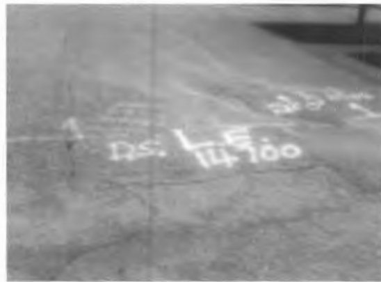
DigSafe Clearance Marks
