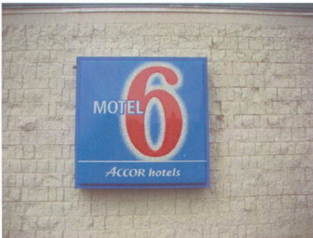
existing conditions for quantity two building signs
