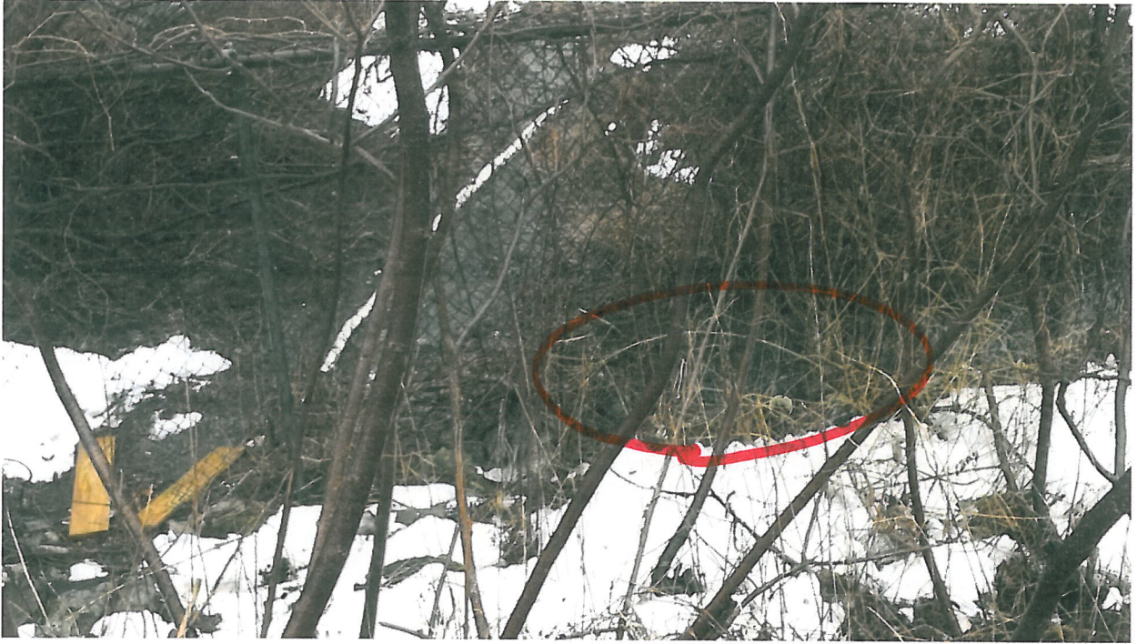
Culvert Outlet Area
