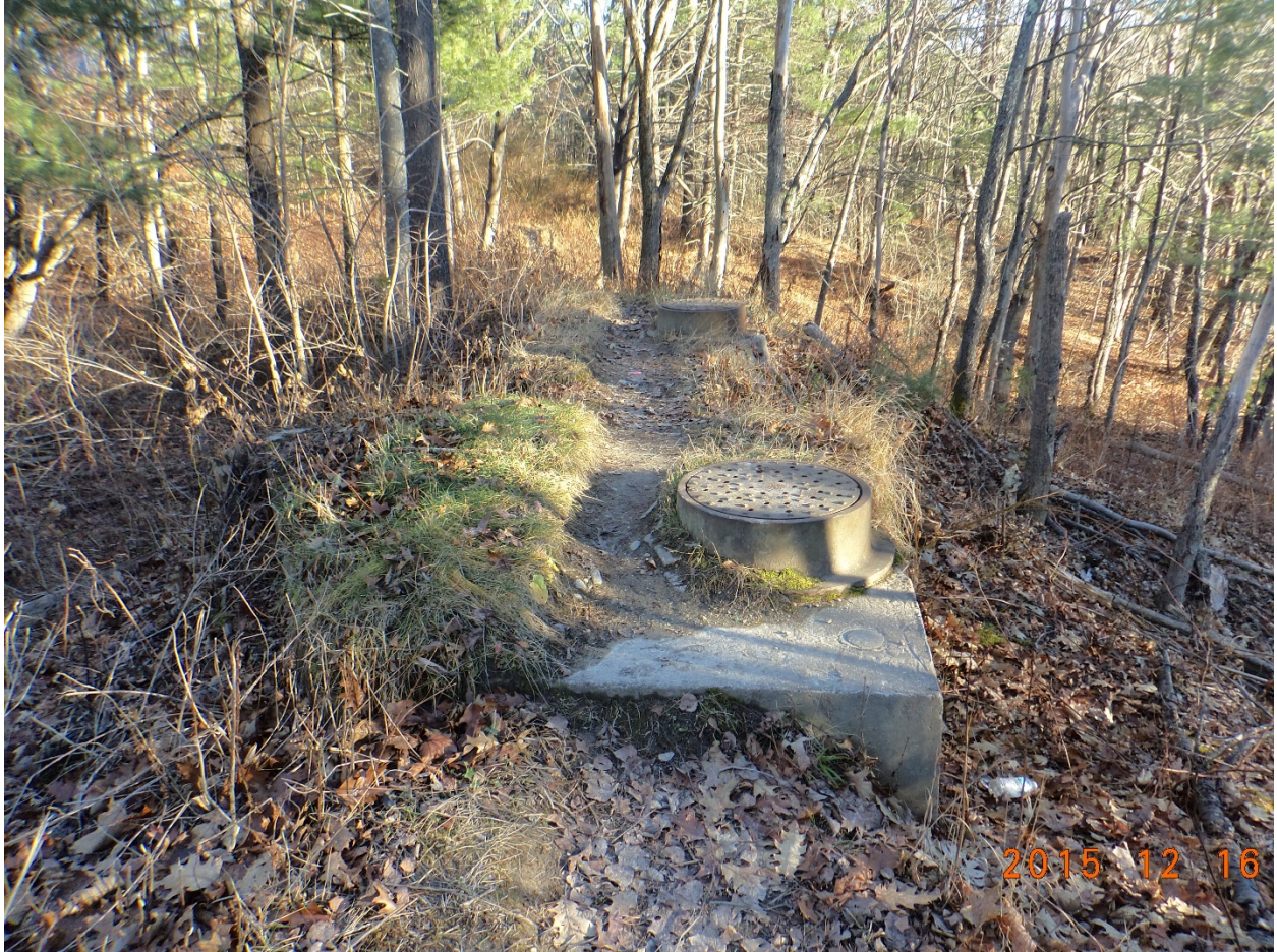
Photo 5: Fore river sewer interceptor pipe CSO Structure. Access road will be constructed to left. Light clearing will be required to complete the access road.
