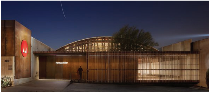
An example of subtle yet strong and beautiful lighting and signage.
