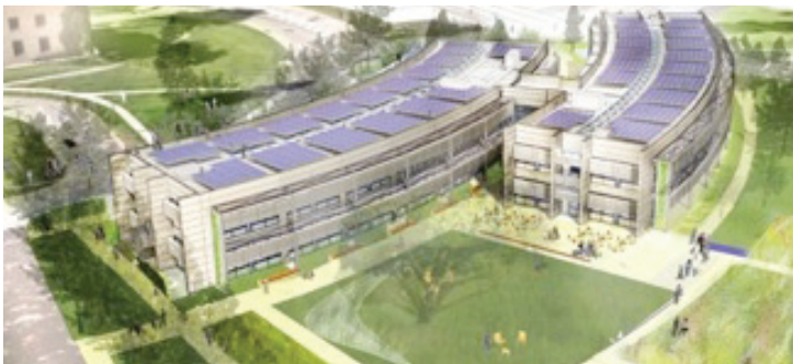
Rooftop photovoltaics can offset the building's energy consumption and put energy back into the grid. -NASA Sustainability Base by McDonough + Partners
