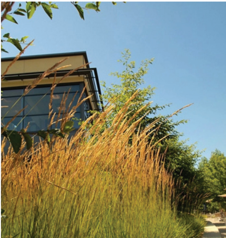
Horizontal sunshading reduces solar gain and planting softens and cools the hard surfaces of the pedestrian walkways and parking.
