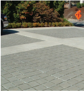
Examples of pervious pavers.
