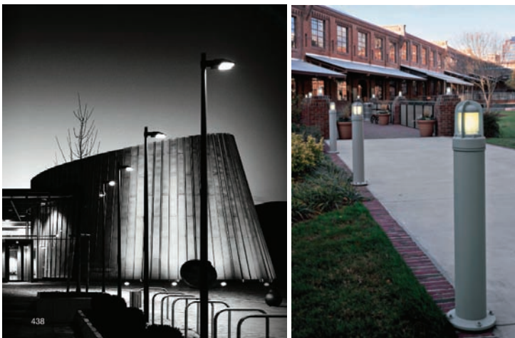
Pedestrian walkways should be lit with bollard type fixtures (right) and parking areas should be lit with pole mounted down-lights (left).
