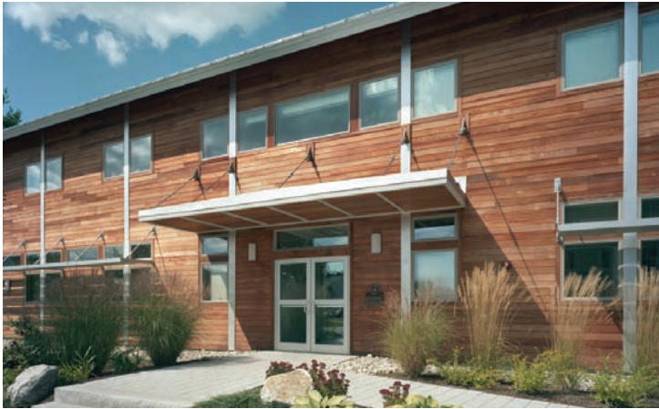
Natural wood siding can provide a great sense of warmth in combination with metal roofs, structure and sun shades. A dynamic and beautiful landscape grounds the building and enlivens the pedestrian edge. -Cascon Headquarters in Yarmouth, ME by Scott Simons Architects
