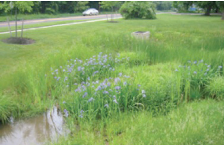
Stormwater treatment wetland, Photo Courtesy of Stormwater Magazine.
