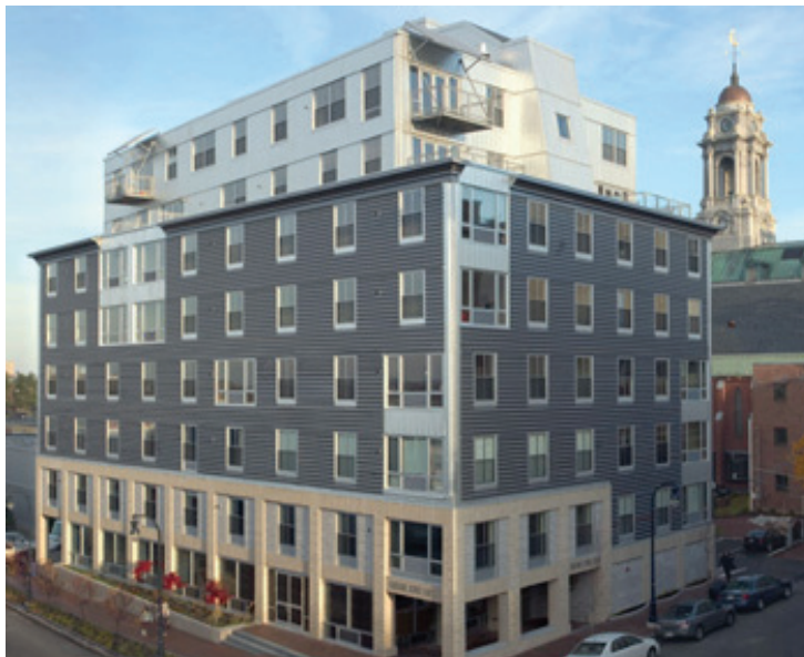
The Chestnut Street Lofts in Portland by TFH Architects blends corrugated metal cladding with rich masonry for a high quality exterior envelope. Careful detailing is essential to make this successful. Note calm and cohesive color palette.
