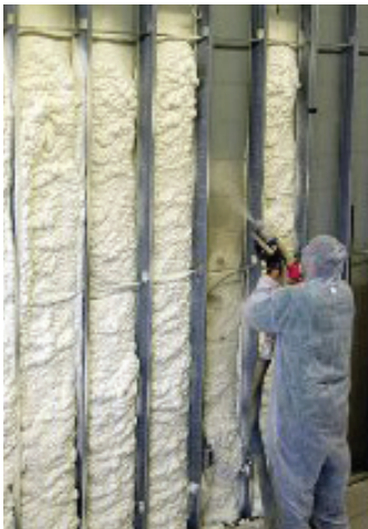
Spray foam insulation creates a tight thermal envelope with minimal air leakage.
