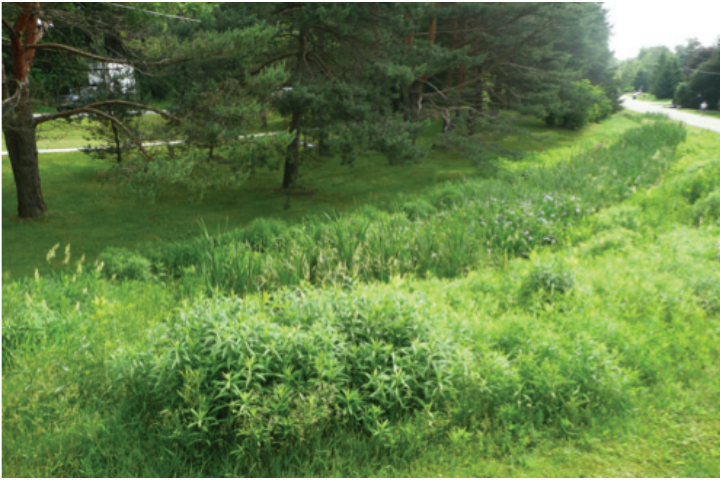
Planted gravel wetlands along the road edge will serve to capture and filter runoff and the native trees and landscape will be largely preserved.
