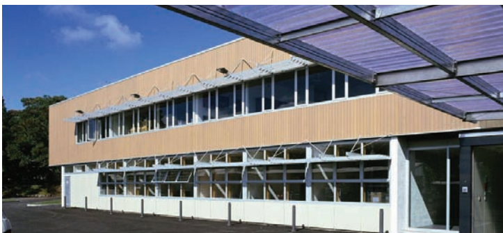
An office building example in Auckland, NZ by Architectus uses operable windows and solar shading devices to naturally control the indoor air quality.
