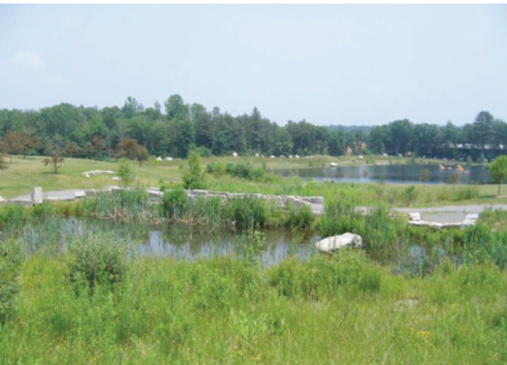
Constructed wetland for stormwater treatment; Town of Acton, MA; design by Woodard & Curran Inc.
