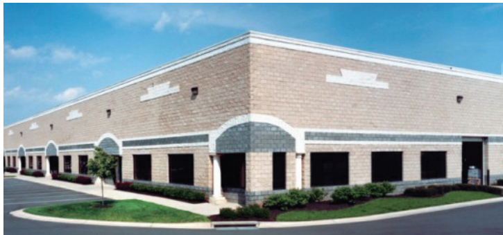
The use of split face CMU such as in this generic building is not allowed. Note lack of relationship to the local climate and built environment.
