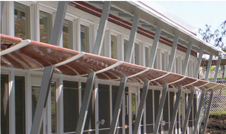
Buildings should be situated appropriately in the landscape with the long side facing south for passive solar opportunities. Solar shading devices in this building at USM Gorham prevent overheating in the summer while allowing for the sun to enter in the winter. -University of Southern Maine Childcare by TFH Architects, Gorham, ME
