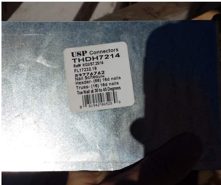
Photo 2: Girder Truss Hanger required (66) face nails
