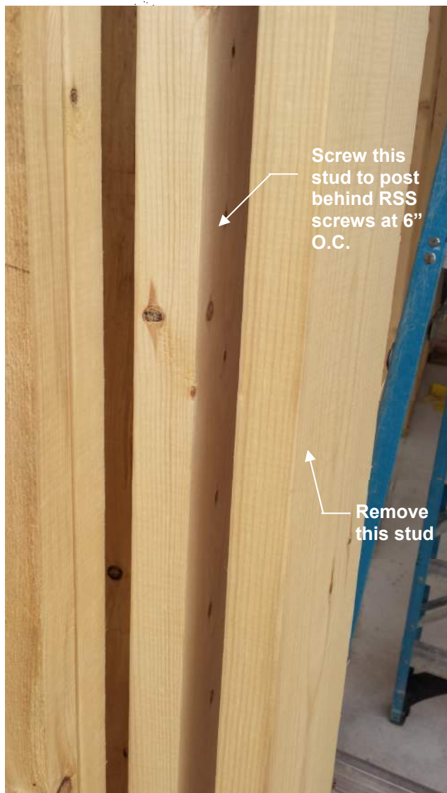
Photo 1: View of Shearwall to Be Fastened to Post Behind with Holddown
