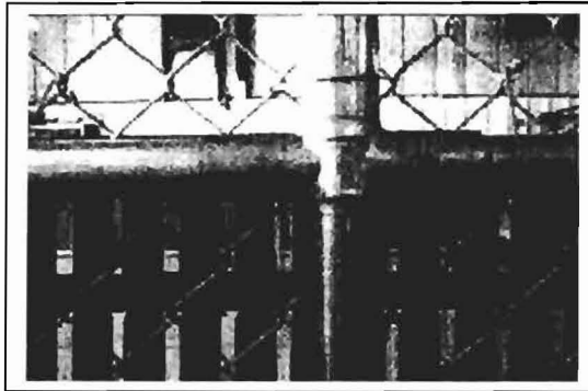
Bolts ground down on all support pole clamps.
