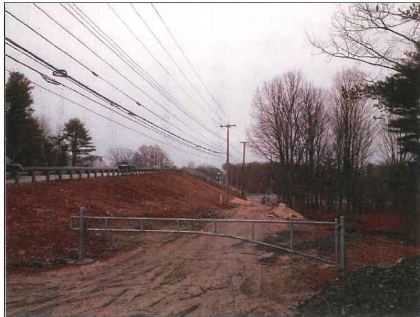
PHOTO 2 – Unltd Gas Regulator off Congress Street
