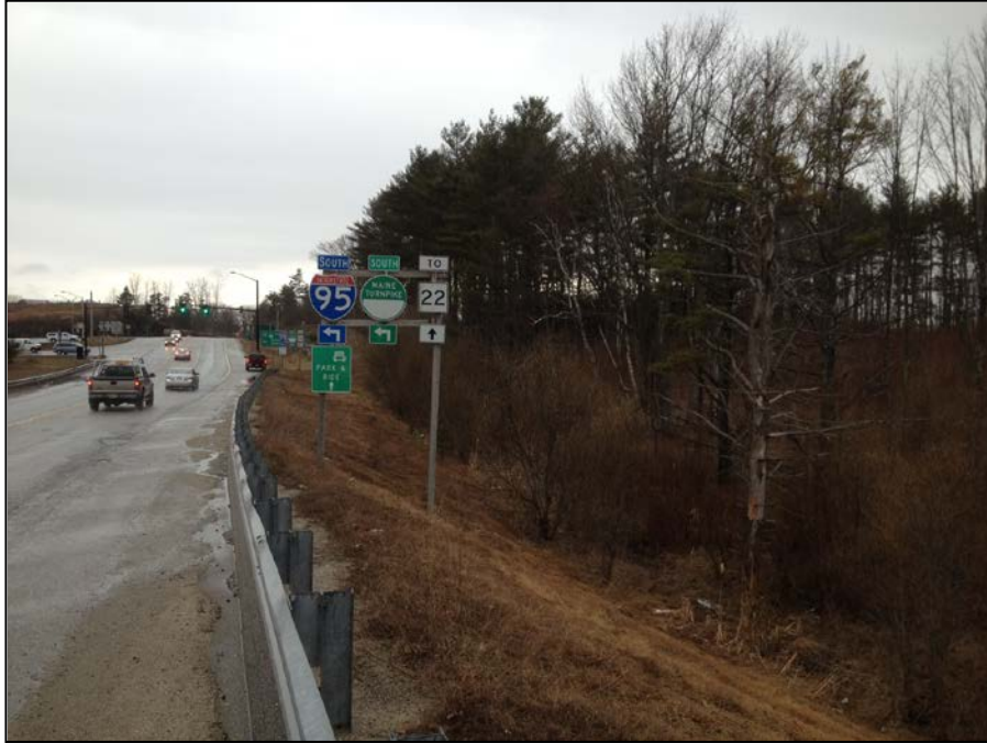
PHOTO 1 – Skyway Drive – West
