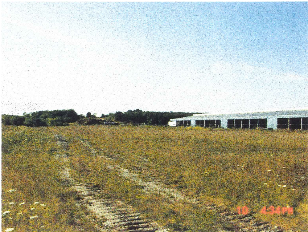
PHOTO LOOKING NORTHWEST AT WEST END OF EXISTING BUILDING.
