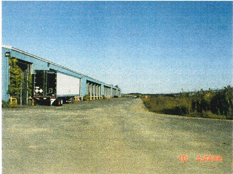
PHOTO LOOKING EAST ALONG SOUTH SIDE OF EXISTING BUILDING AT AREA OF PROPOSED PAVEMENT WIDENING.
