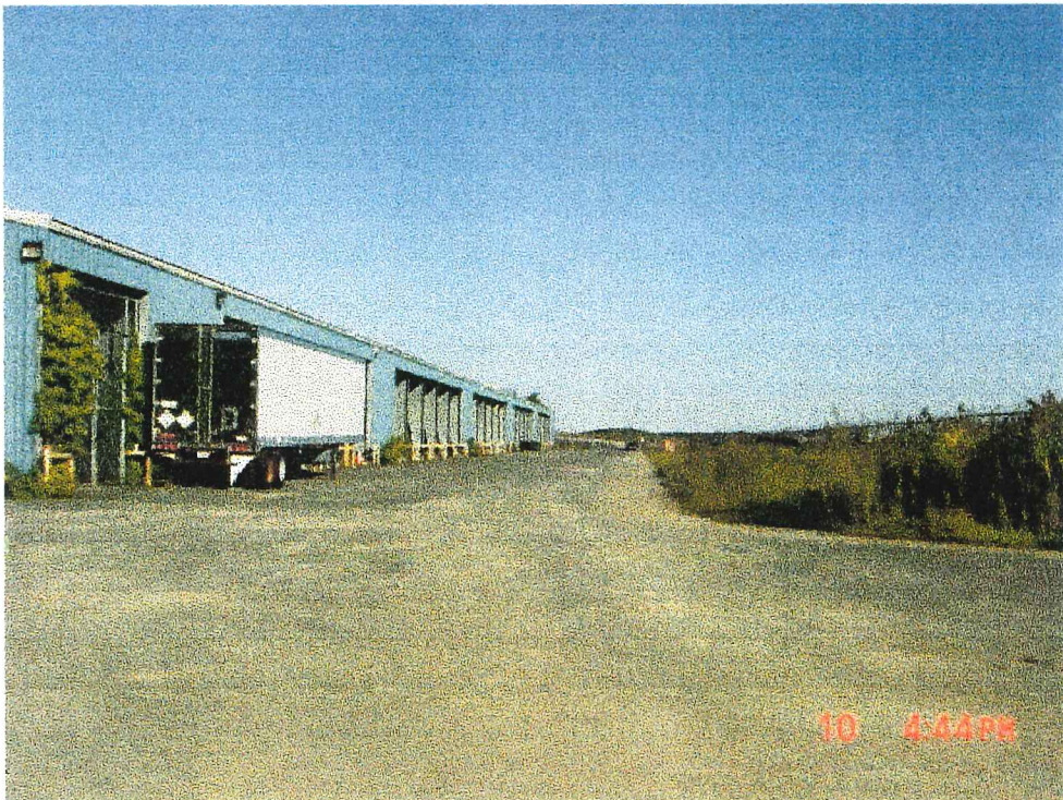
PHOTO LOOKING EAST ALONG SOUTH SIDE OF EXISTING BUILDING AT AREA OF PROPOSED PAVEMENT WIDENING.
