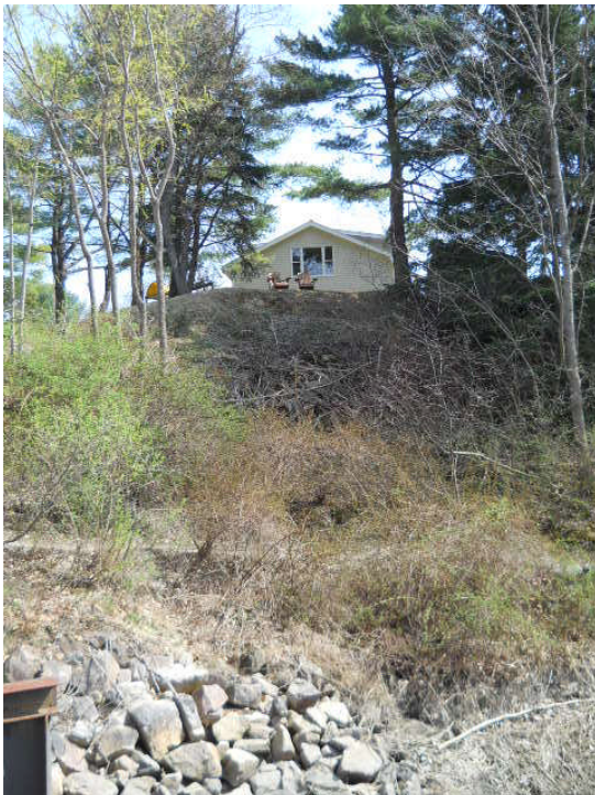
Photo 6. Proposed pipe run to outfall southwest of 81 Winding Way (proposed outfall just right of existing rip rap)
