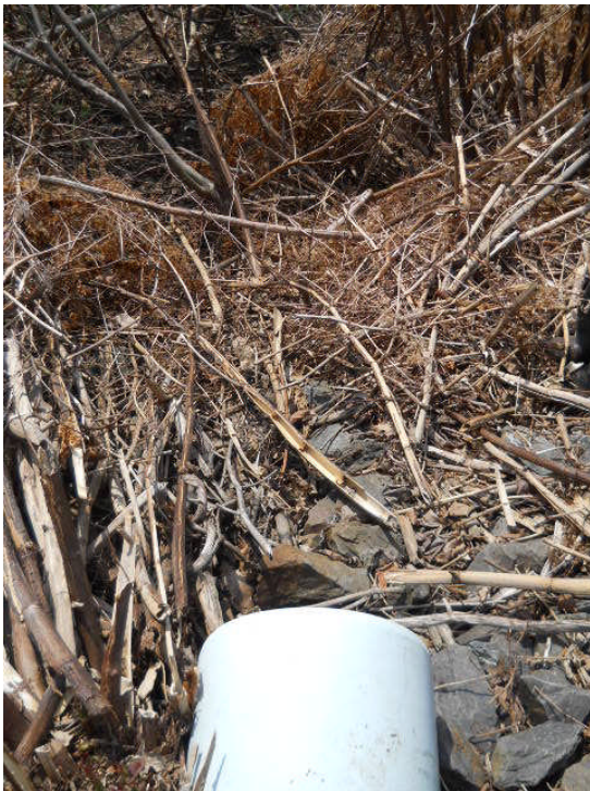
Photo 8. Existing outfall to receive riprap located northwest of 73 Winding Way
