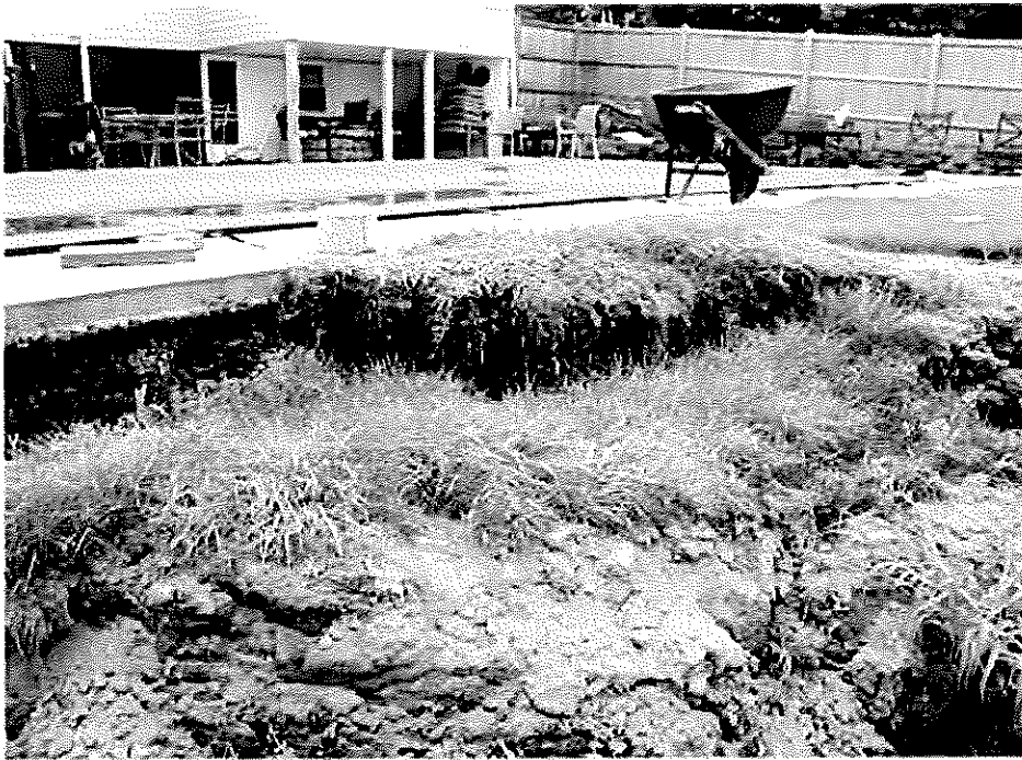
Photo 5. Project Need – Stabilize the slope failure condition (Surface Tension Crack behind house #81)
