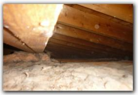
The hip rafters and ridge are 2x8 lumber. A double 2x8 is installed below the ridge and appears to be supported by two 4x4 posts (photos below). The support below the 4x4's was concealed.
