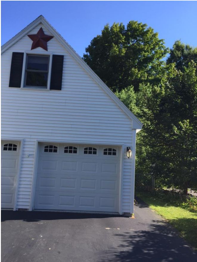
Photos of 1375 Westbrook Street Garage Exterior
