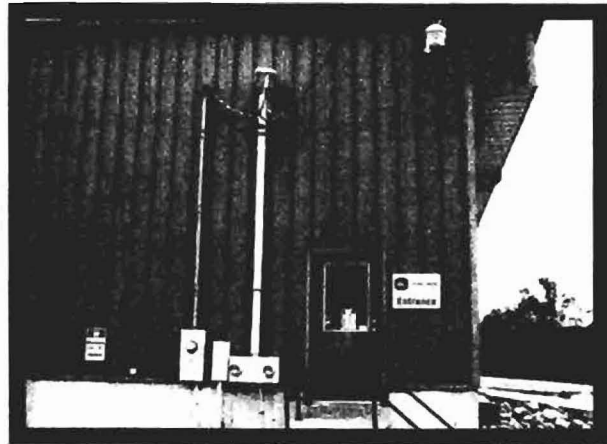
LEFT SIDE OF BUILDING
