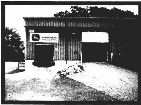
FRONT OF BUILDING
