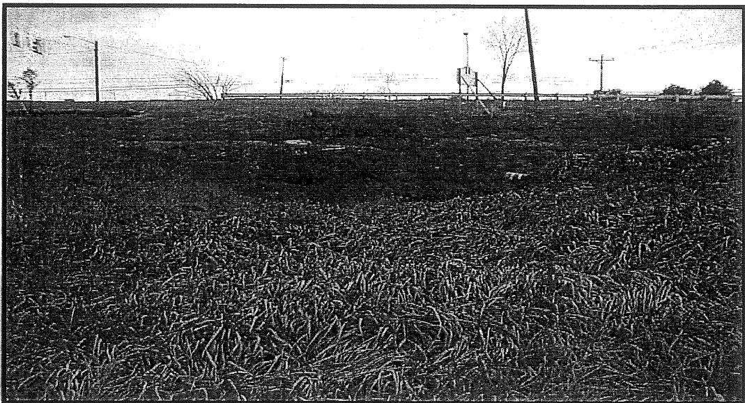
A WELL STABILIZED VEGETATED SWALE SHOWS LITTLE SIGN OF EROSION VELOCITIES OR FLOWS. THIS SWALE ALSO FUNCTIONS AS A POND SPILLWAY
