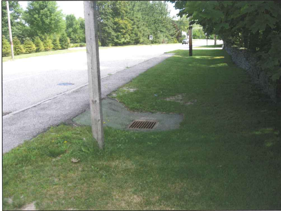
View of existing catch basin off Johnson Road
