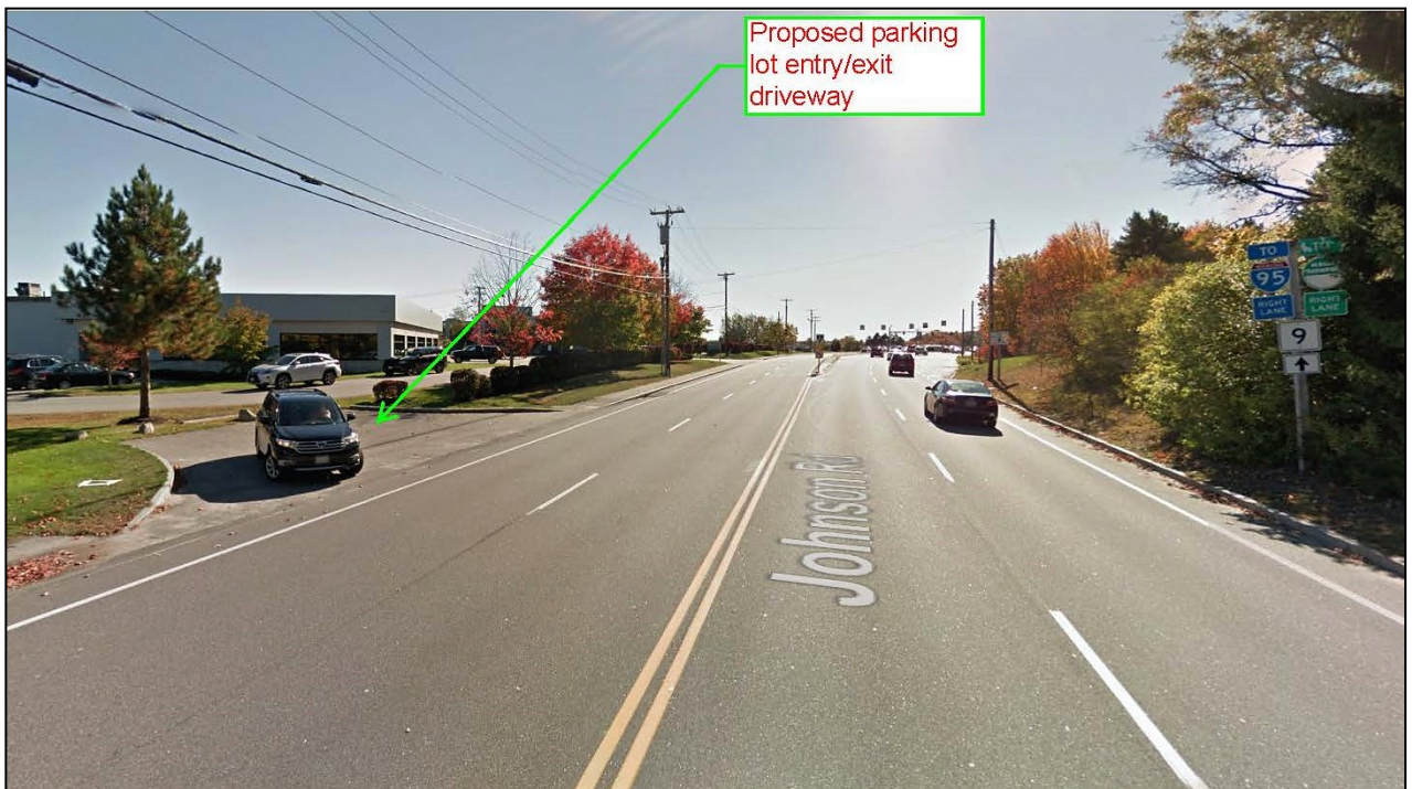
Existing Curb Opening on Johnson Road
