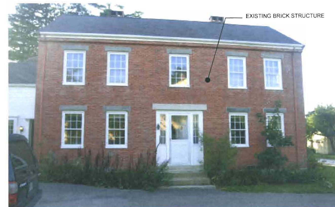
SITE PHOTOGRAPH (EAST ELEVATION)
