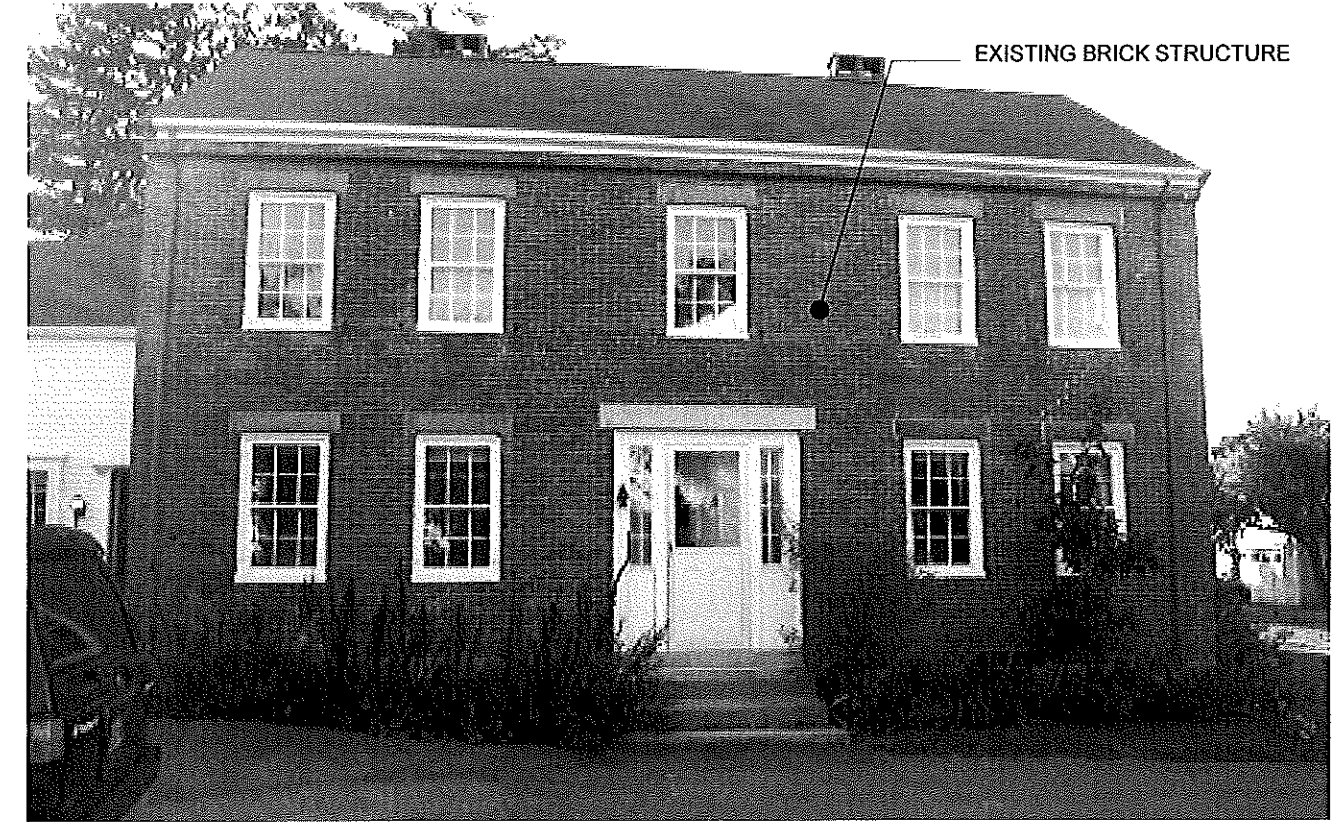
SITE PHOTOGRAPH (EAST ELEVATION)
