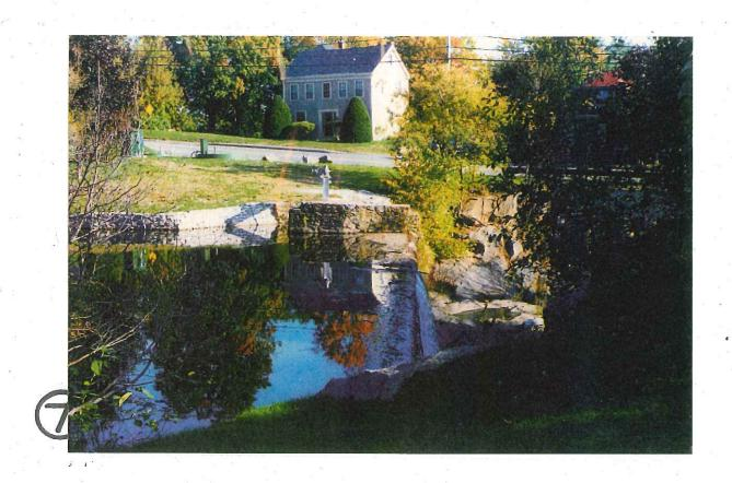
7. View looking north across Stroudwater Dam. The drop at dam is 15-20 feet. Proposal is to add an iron railing (2 ½" diameter, 3 'high, 10 to 12 feet long) for safety. Railing is to be drilled into rock outcrop in foreground of photo.
