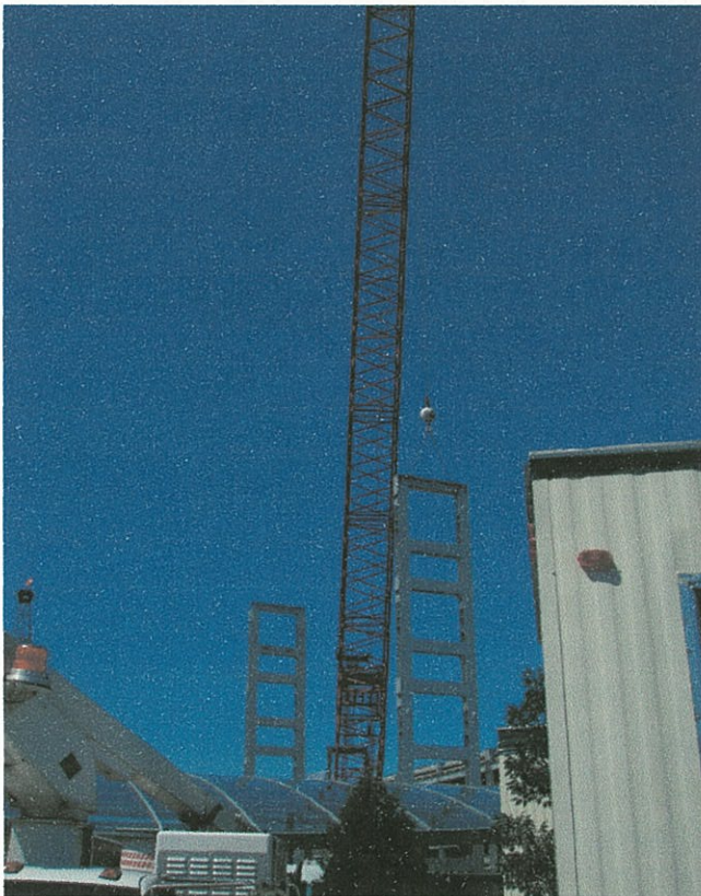
Installation of H Frame G/13
