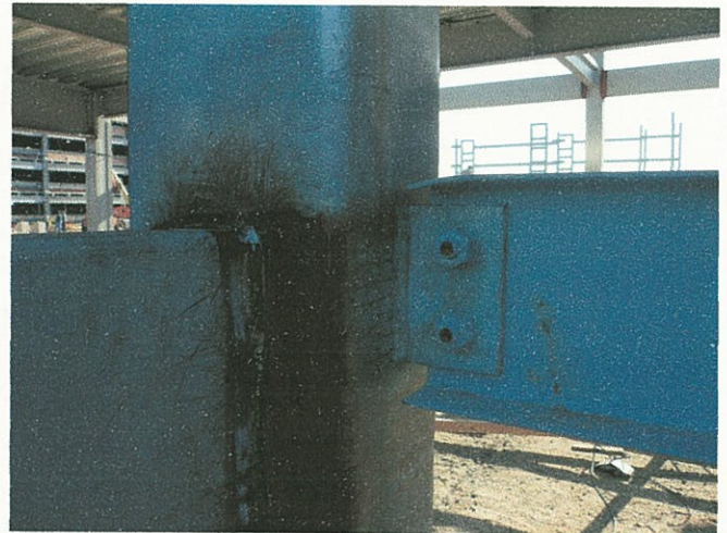
W8x10 landing beam (right) and HSS flight header (left). The W8x10 was raised 2".
