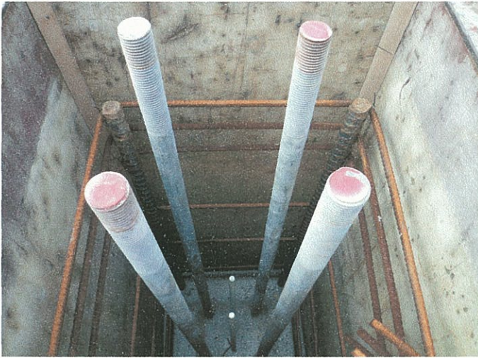
Pier F/9 Reinforcement
