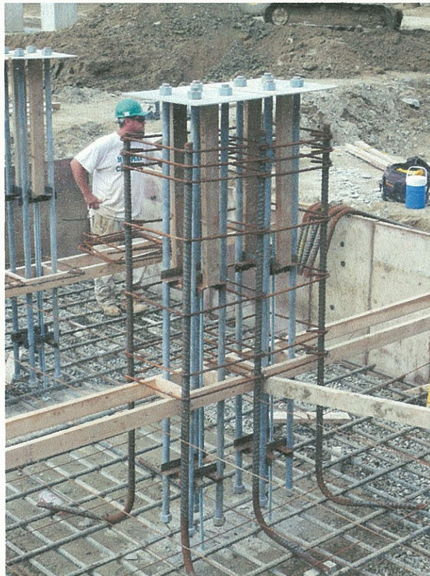
Pier Reinforcement @ F/6-7 footing
