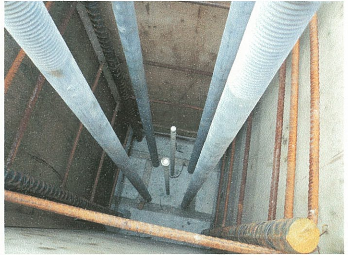
Pier F/8 Reinforcement
