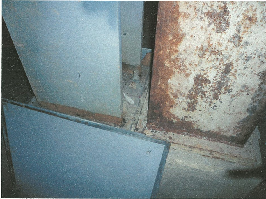
Offset columns @ E.1 line w/ 3/8" plate
