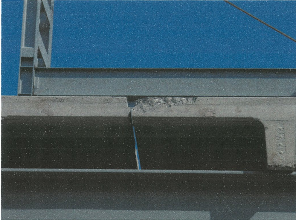
Damaged DT Flange
