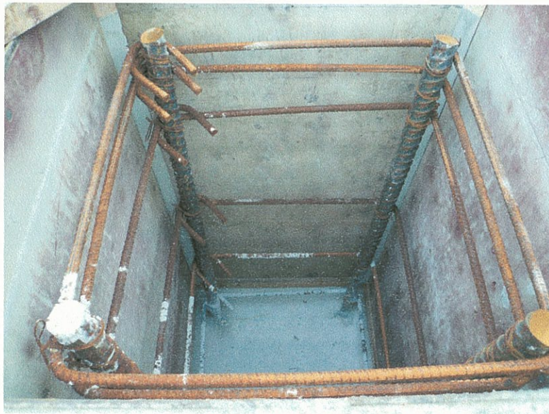
Reinforcement for Canopy Pier RD/12
