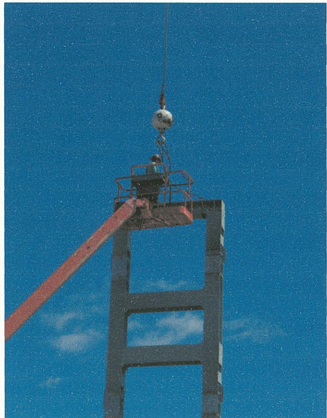
Detaching Crane from Frame
