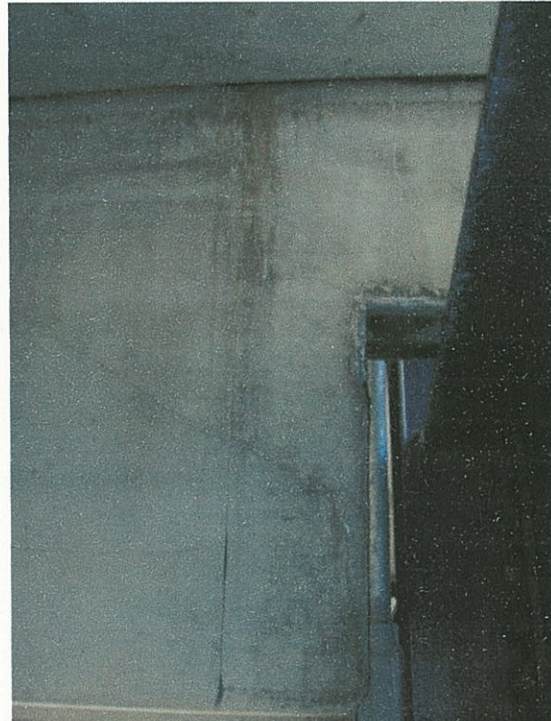
Phase 1 DT – Cracks at Dapped Ends
