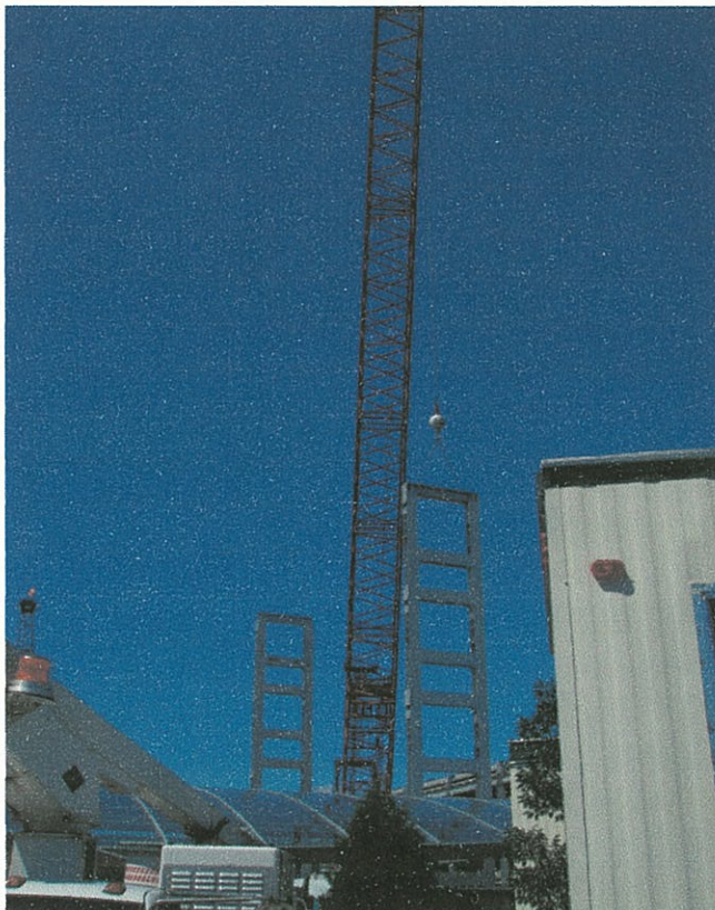
Installation of H Frame G/13
