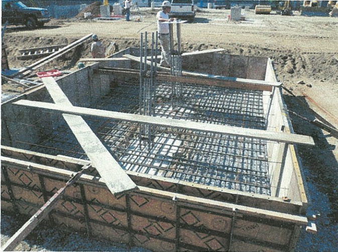
Garage Footing F/11 Reinforcement
