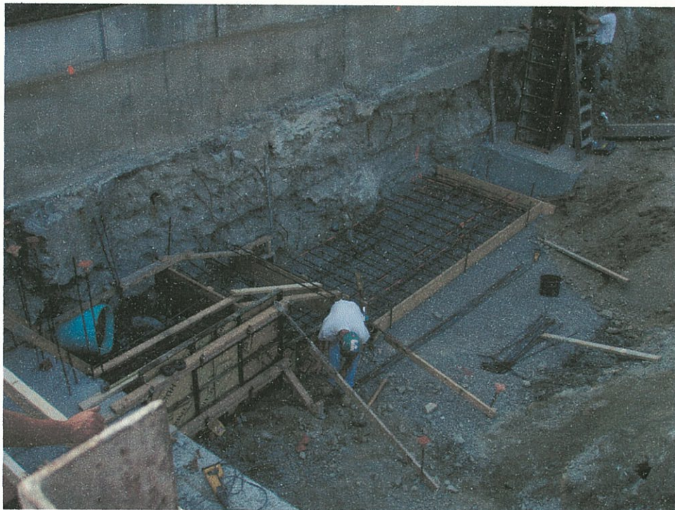
Vault Stair Footing
