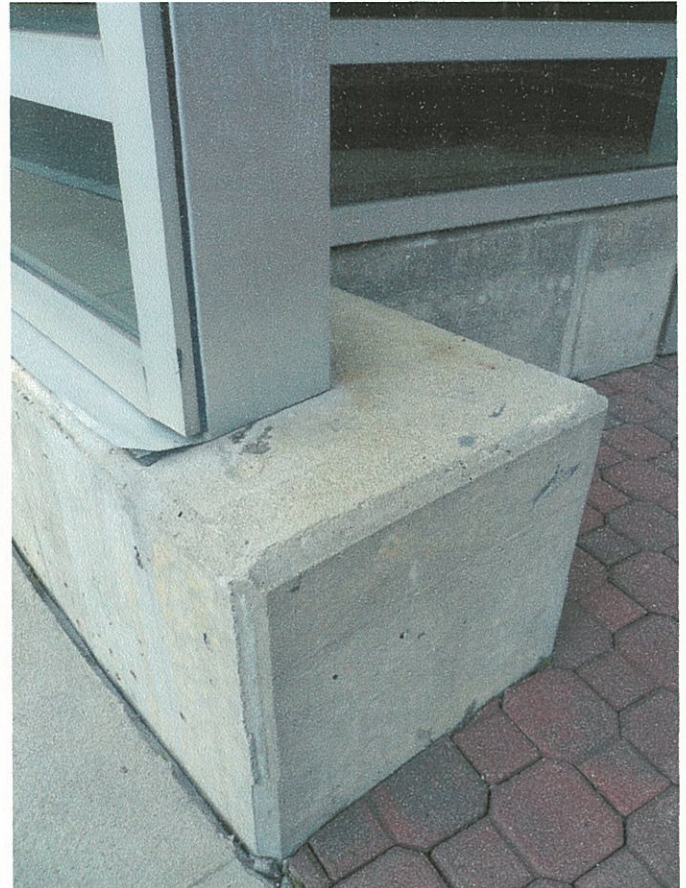
Foundation wall @ existing East Stair Tower
