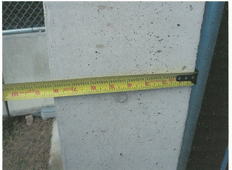
Field measurement – precast wall thickness
