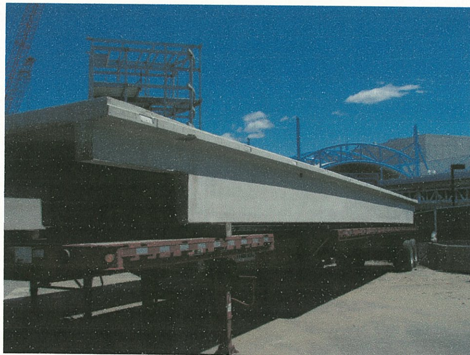
First DT Delivered to Site
