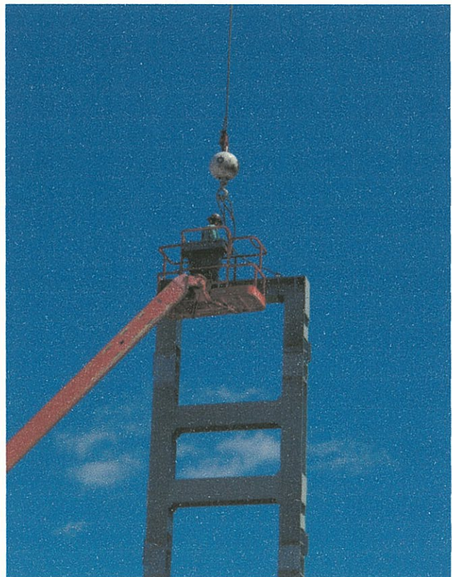
Detaching Crane from Frame
