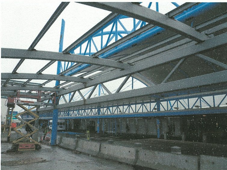
Southeast Transitional Canopy Framing – HSS Truss
