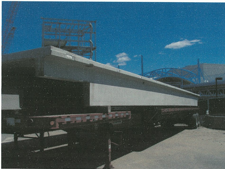
First DT Delivered to Site
