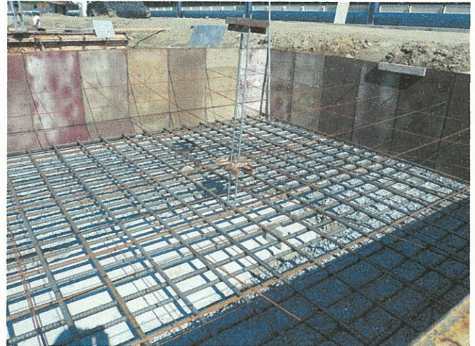
Garage Footing F/10 Reinforcement
