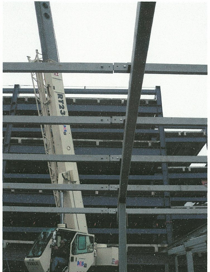
C6 channel splices 1'-0" west of grid 11.6
