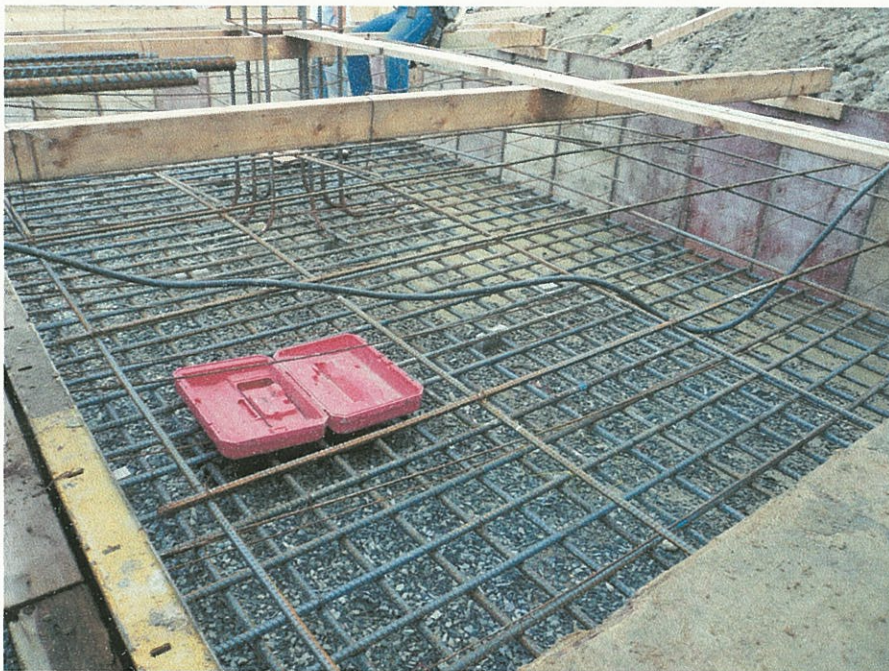
Footing F/12-13 reinforcement
