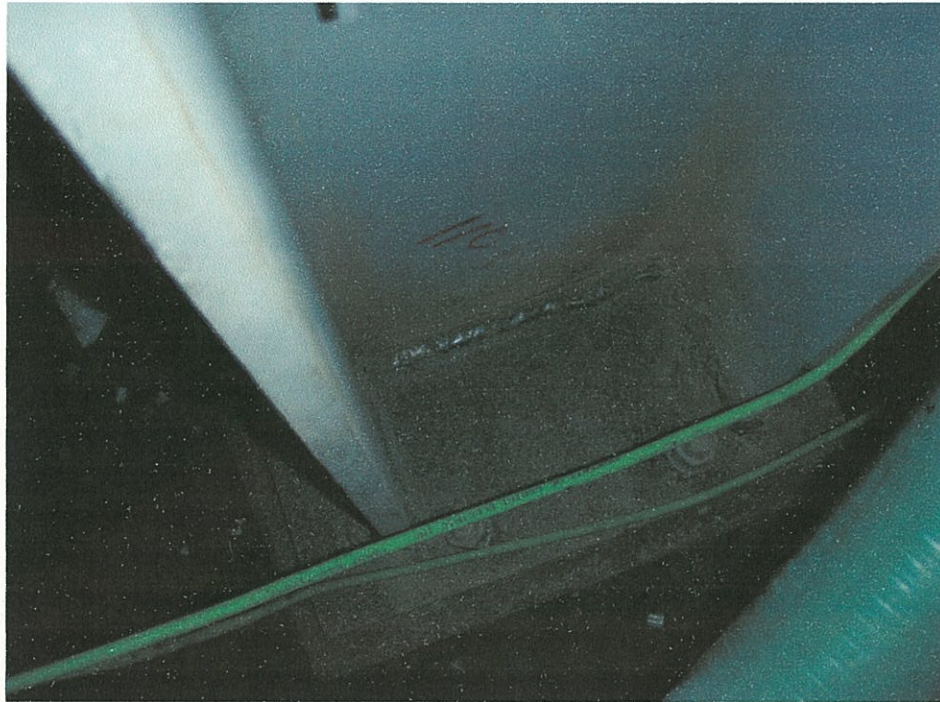
Weld of Column to Base Plate E.1/12
