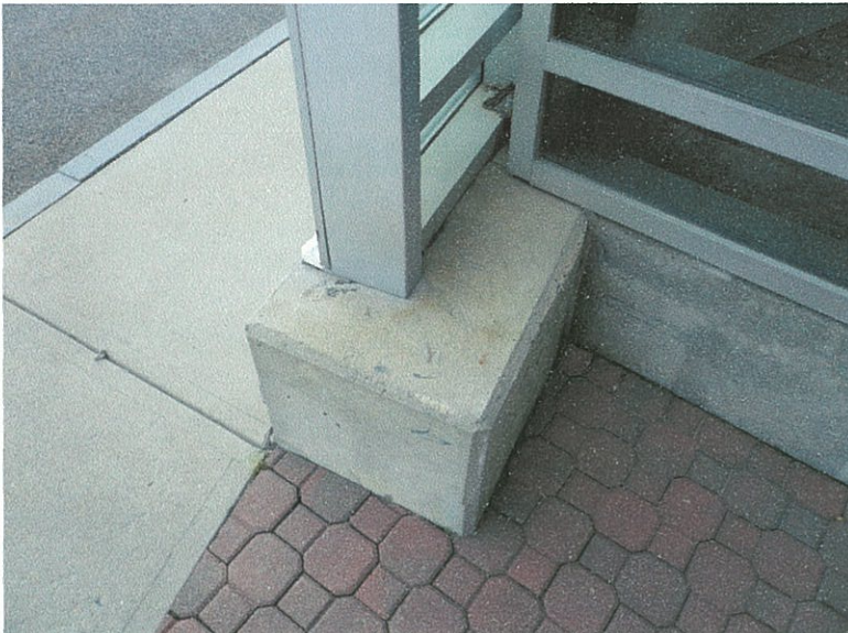
Foundation wall @ existing East Stair Tower
