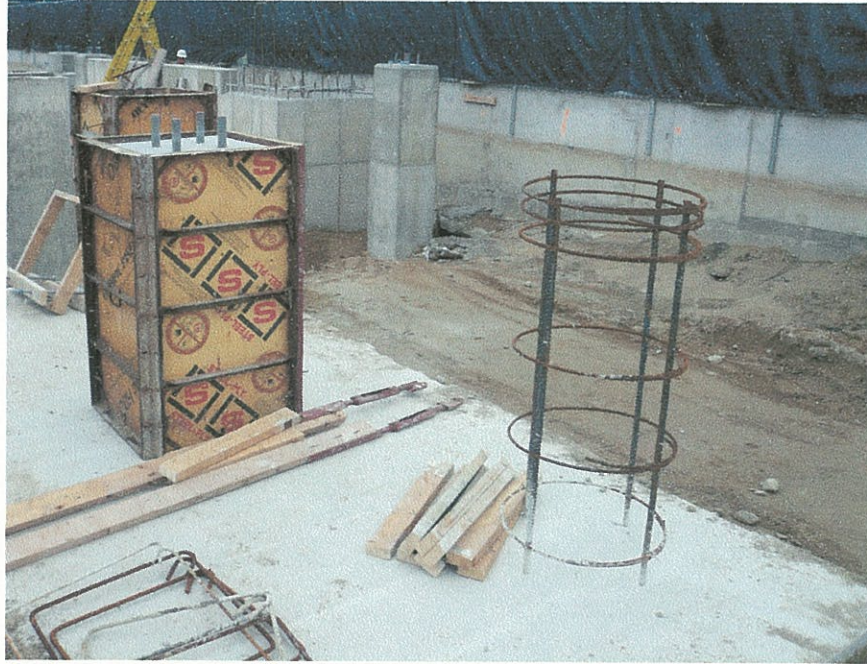
Garage Pier H/11.9 (left) and Canopy Pier RC/12 (right)
