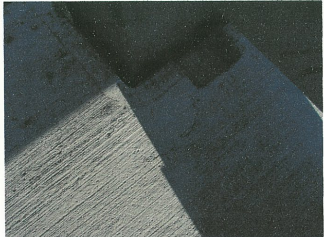
Crack in DT Flange
