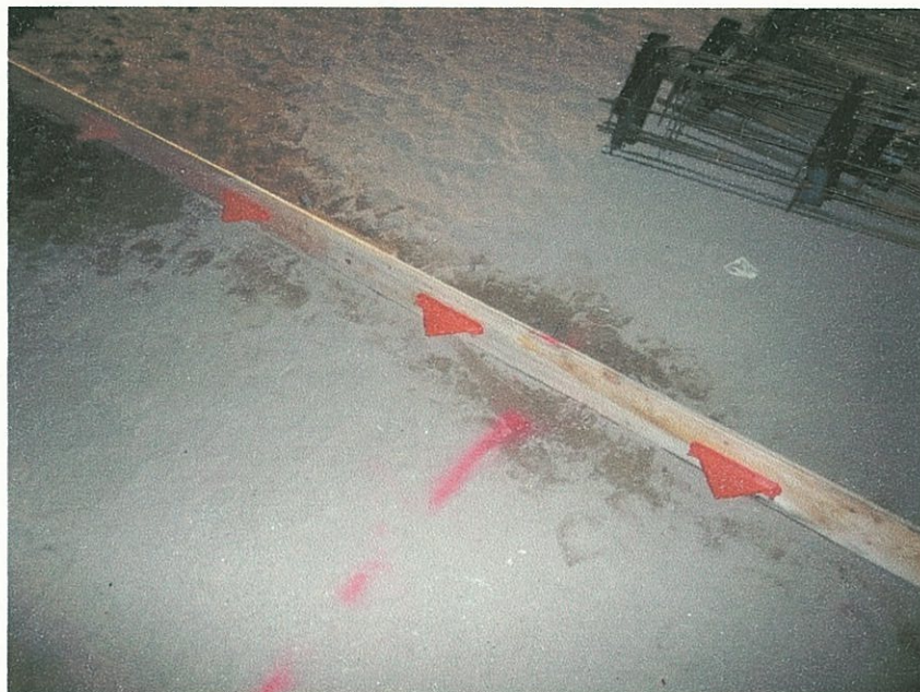
Diamond dowels @ construction joint
