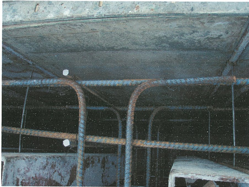
Wall Intersection at T Pier (G/13)
