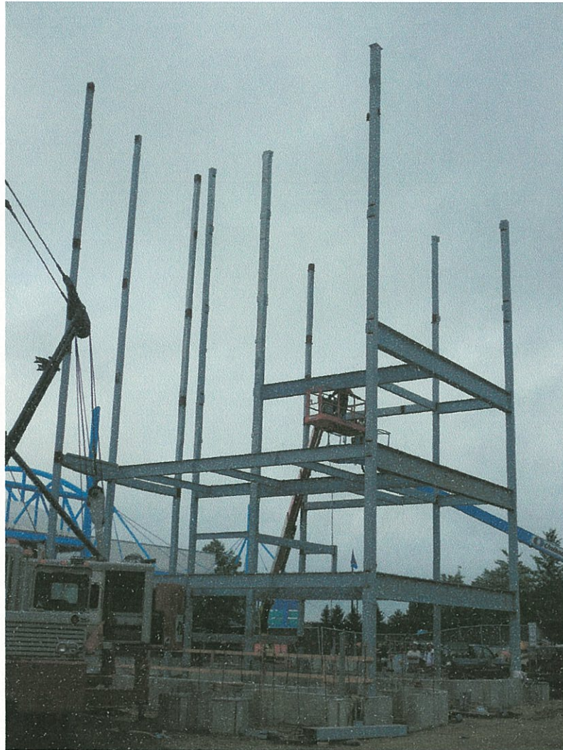
Stair Tower structural steel as of July 23, 2008
