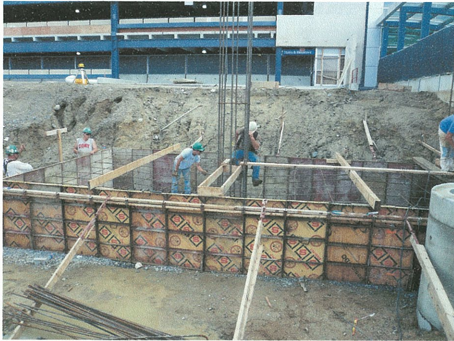
Revised footing F/12-13 near Manhole (far right)
