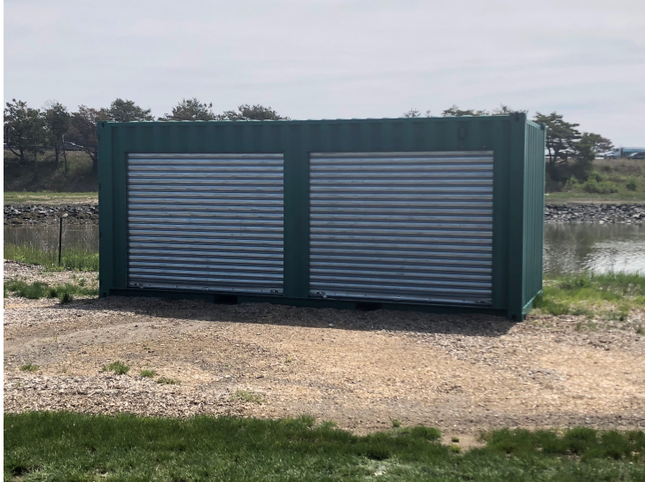
Structure D: Water Station container
