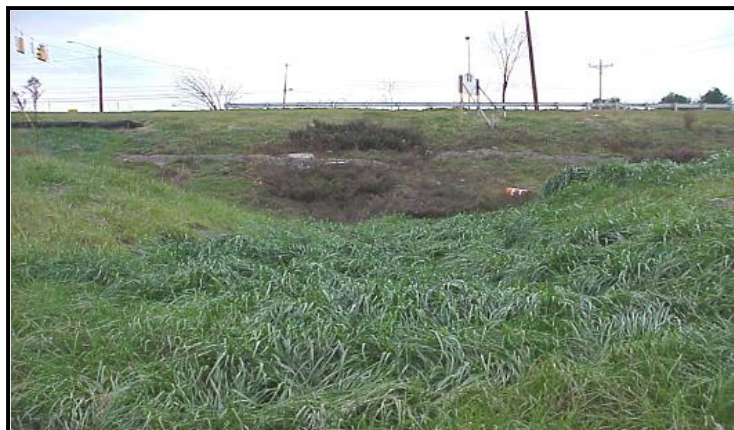
A WELL STABILIZED VEGETATED SWALE SHOWS LITTLE SIGNS OF EROSION VELOCITIES OR FLOWS. THIS SWALE ALSO FUNCTIONS AS A POND SPILLWAY
