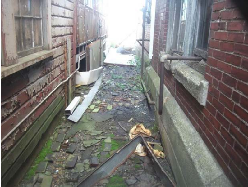
9. Waste potential ACM roof shingles in between Buildings #1 and #2
