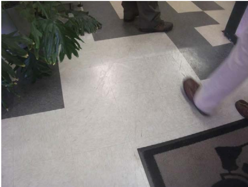
3. Potential ACM floor tile in Building #1, room 1.
