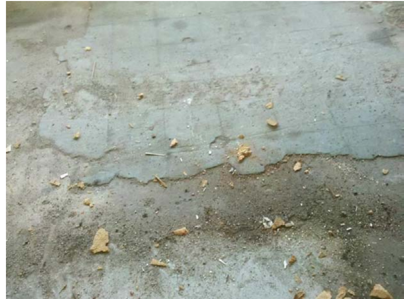
6. Potential ACM floor tile in Building #2, room 1.
