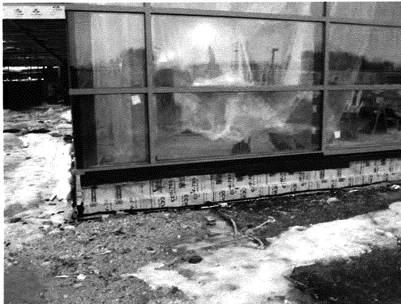
Photo No 2 Test Specimen #2 Exterior View of Specimen with Test Area Highlighted
