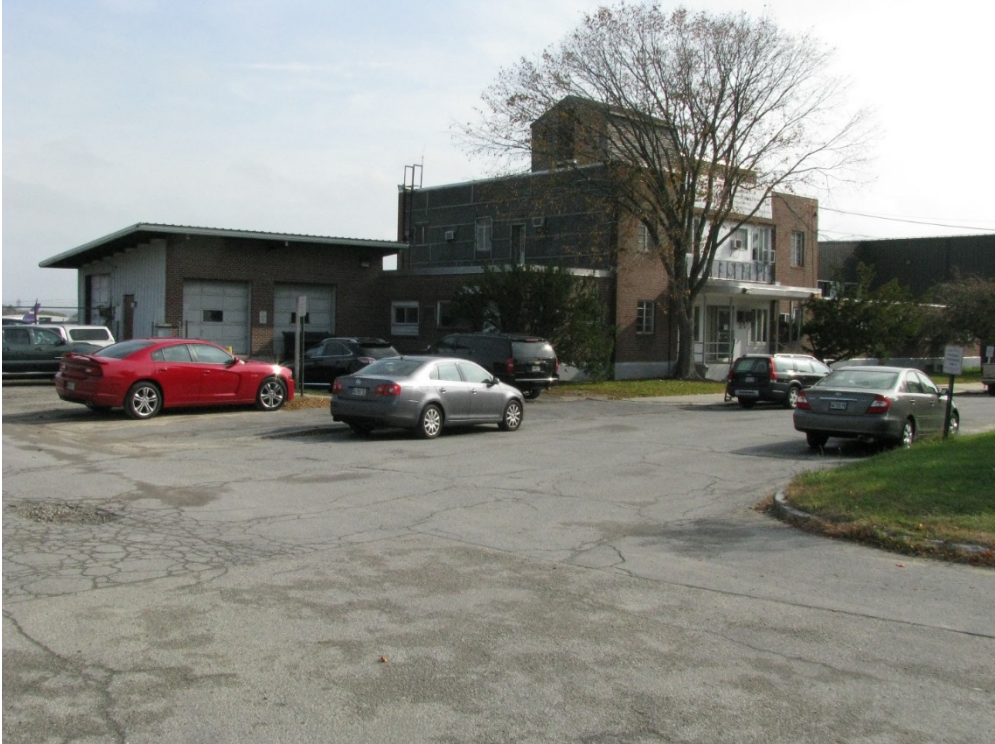
West Side from North
