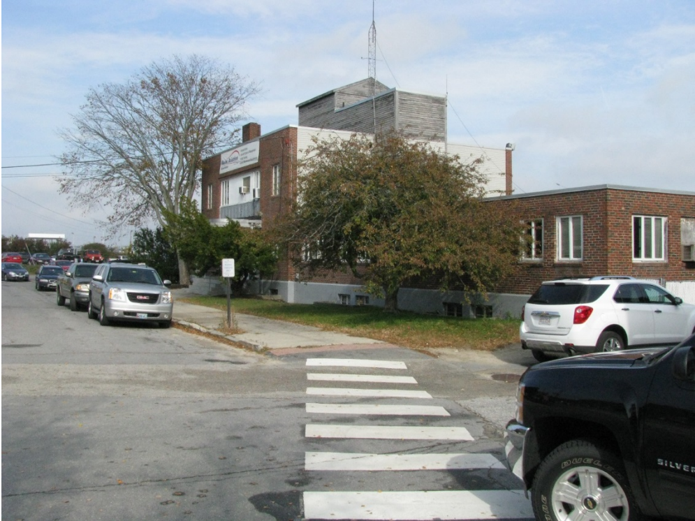
West Side from South
