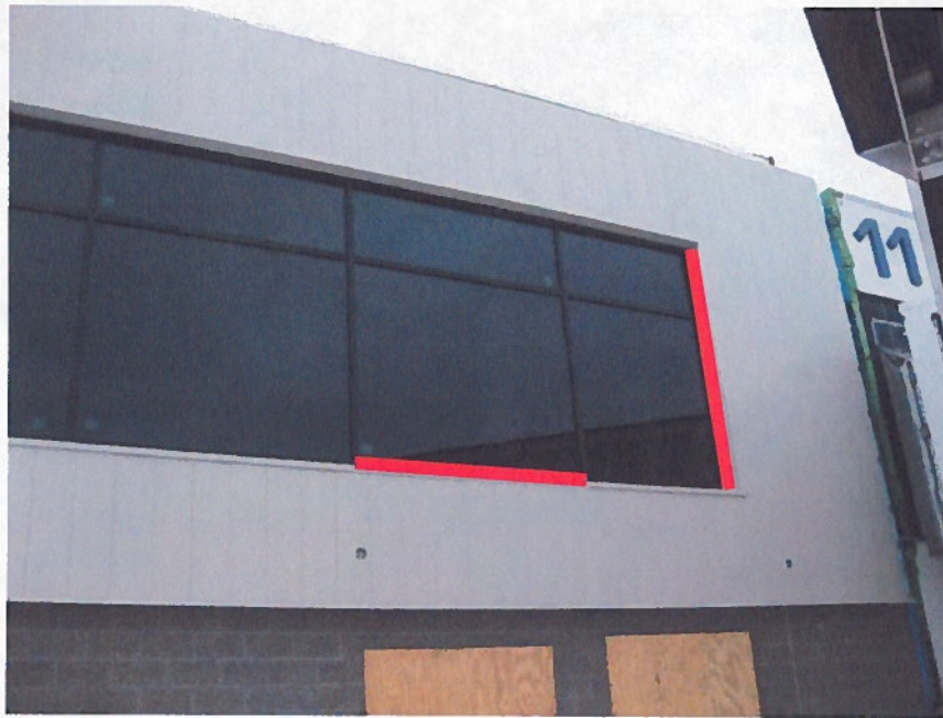
Photo No. 1 Test Specimen #1 Exterior View of Test Specimen with Test Areas Highlighted
