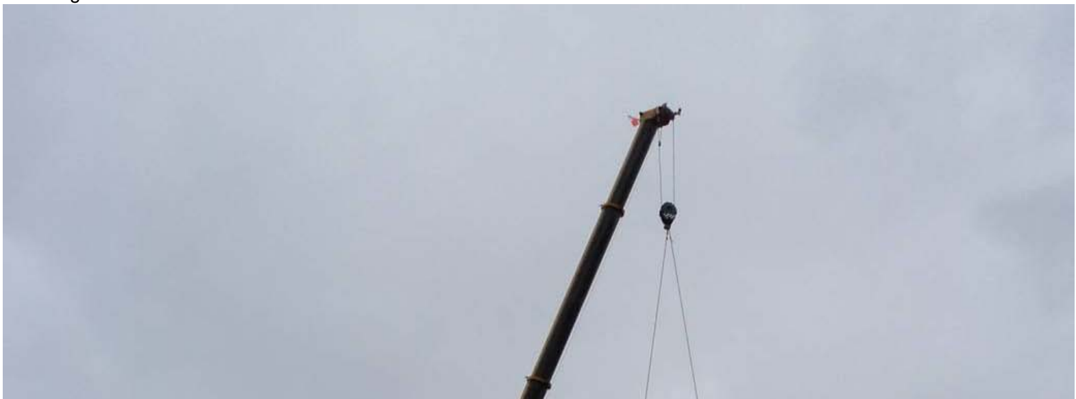
Area C Installing truss section for tower crane
