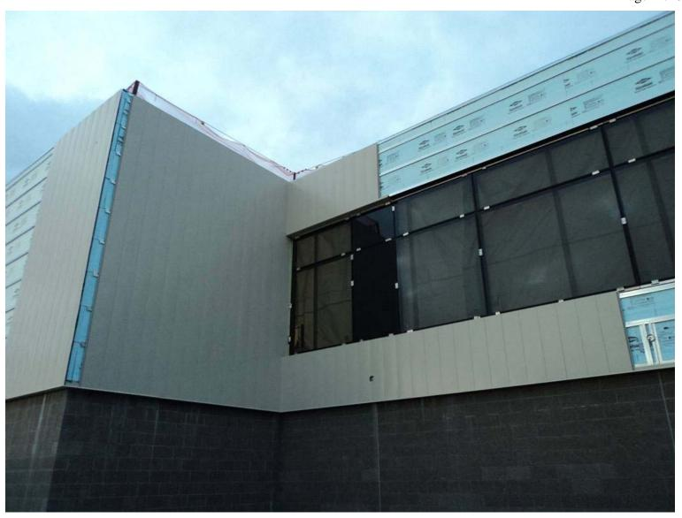
Curtainwall Framing, Dens Glass, and Waterproofing at West Exterior
