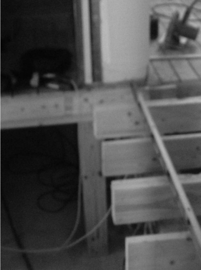
Photo #3 Showing New posting and first floor framing
