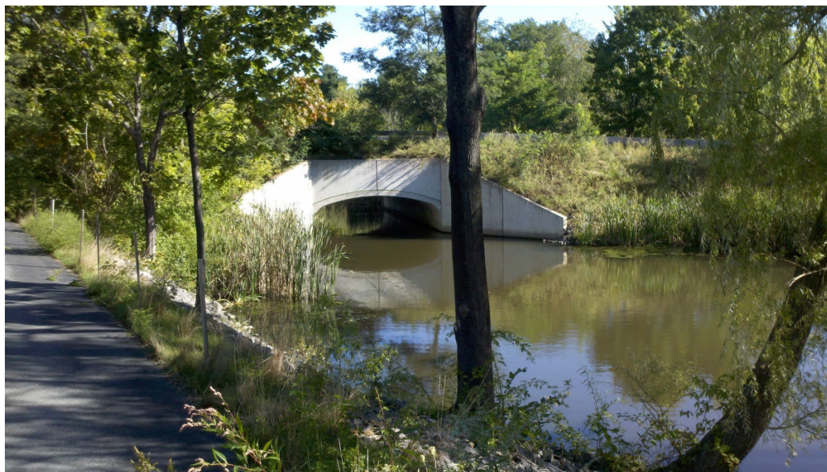
Figure 4-3 View of culvert crossing under Capisic Street, facing northeast (Photo by Woodard & Curran, September 2012)
