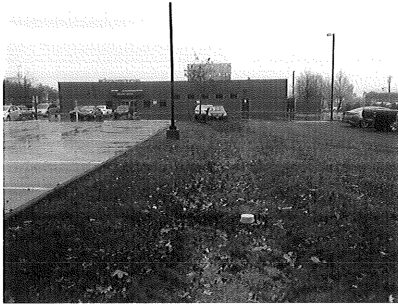
PHOTOGRAPH #3: Underdrained soil filter currently treating the parking lot constructed in 2006
