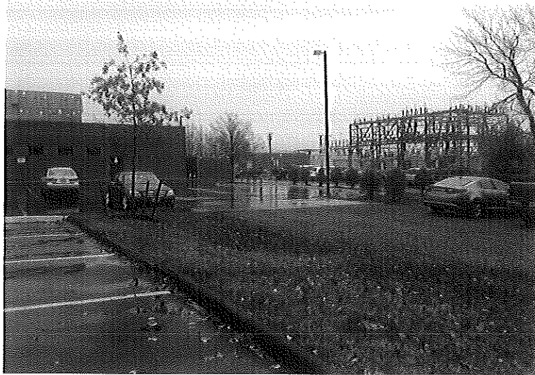
PHOTOGRAPH #1: Existing and proposed parking lots, as seen from tax map lots 24 & 25
